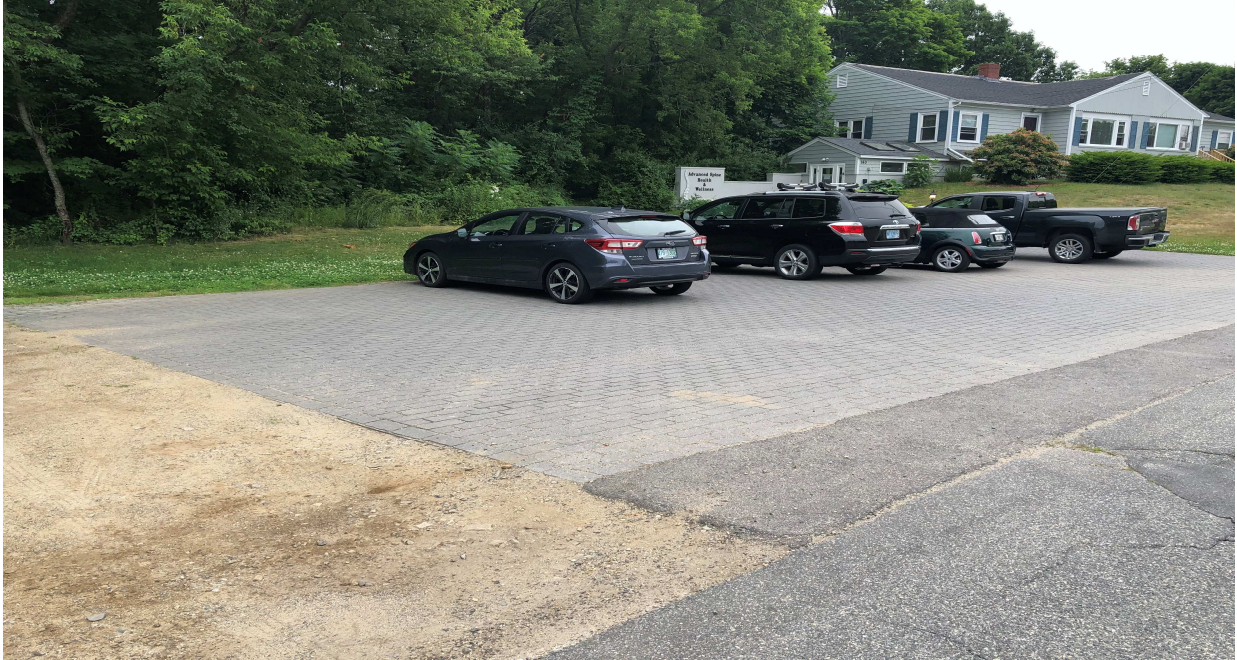
Photo 3: On Edmond Ave looking South towards Pervious Paver parking area and structure.
