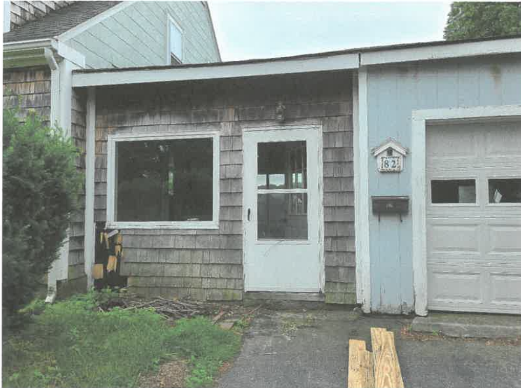
PHOTO 4 - FRONT HOUSE – BREEZEWAY – TO BE REMOVED
