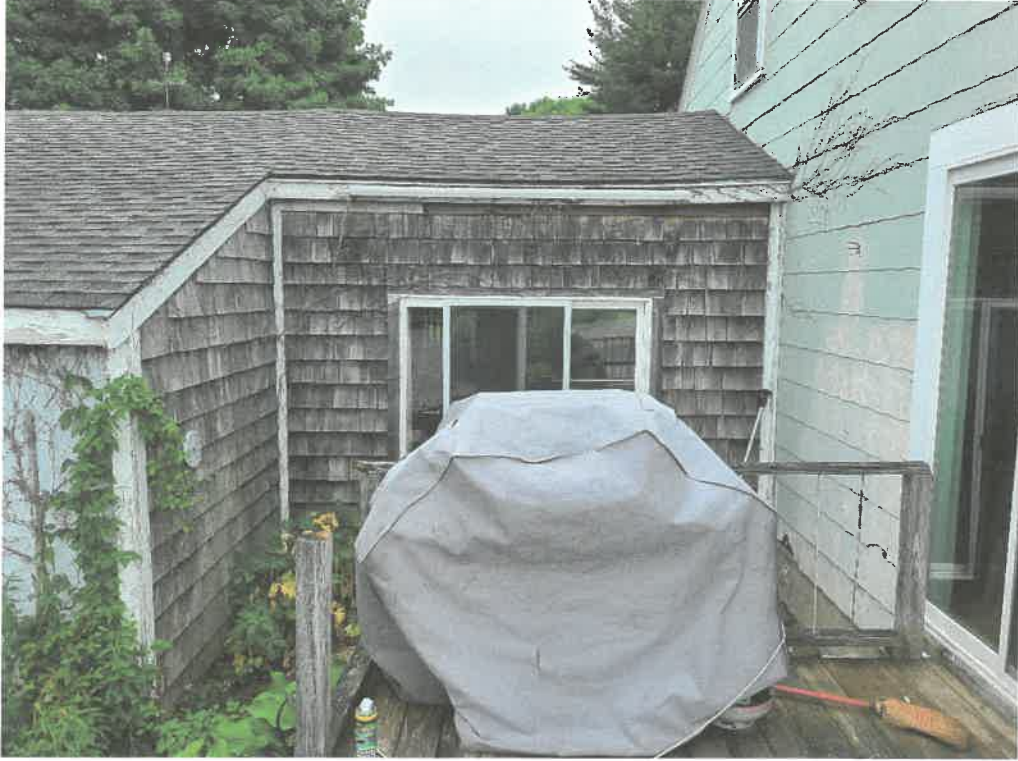
PHOTO 3 - BACK HOUSE - BREEZEWAY – TO BE REMOVED
