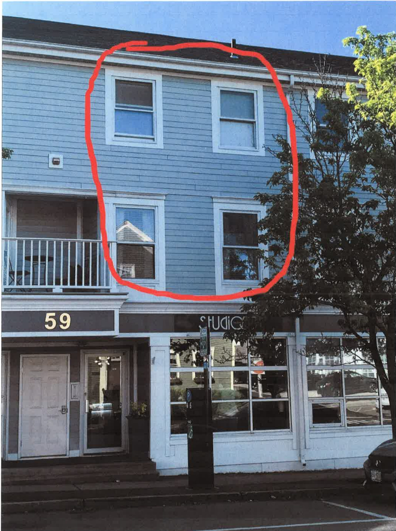
4 windows on Deer Street side to be replaced.
