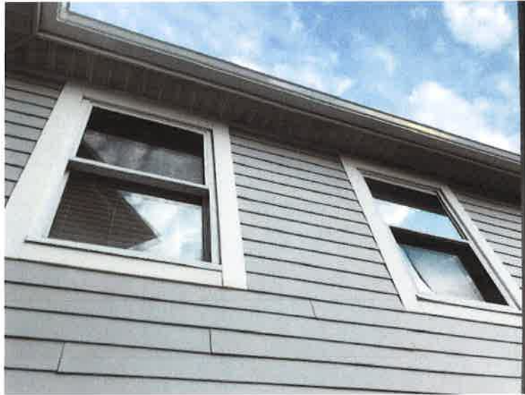
The windows (above) are the existing exterior facing the Sheraton ↗
