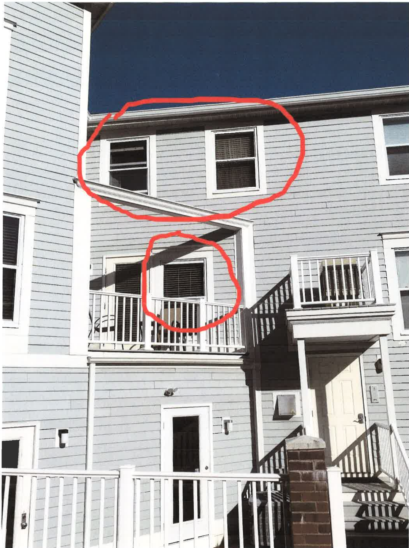
3 windows on sheration side to be replaced
