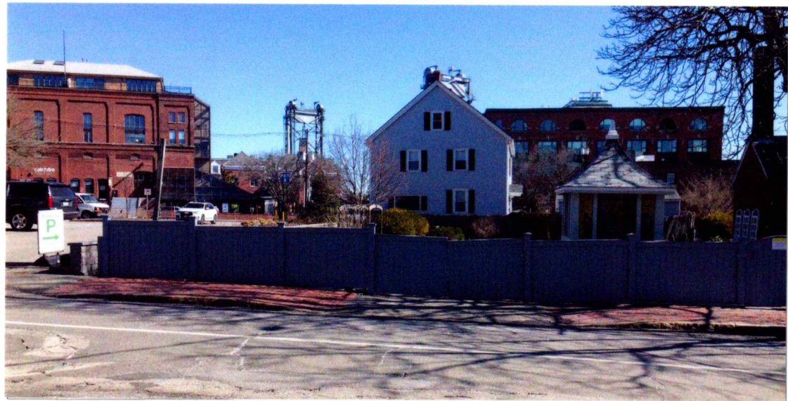
VIEW EAST FROM CHAPEL STREET
