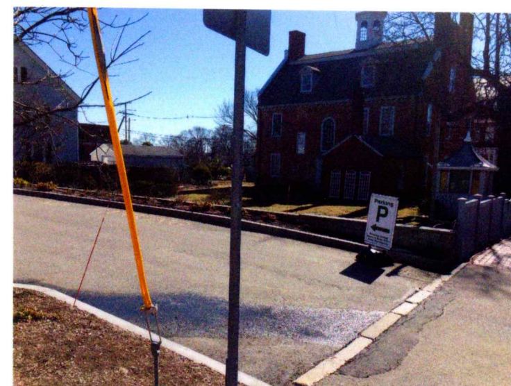
SOUTH VIEW WITH EXISTING RETAINING WALL
