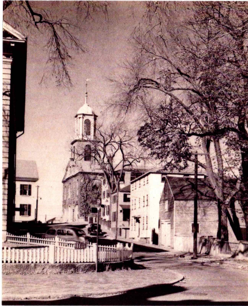
PHOTO OF ORIGINAL CARRIAGE HOUSE
