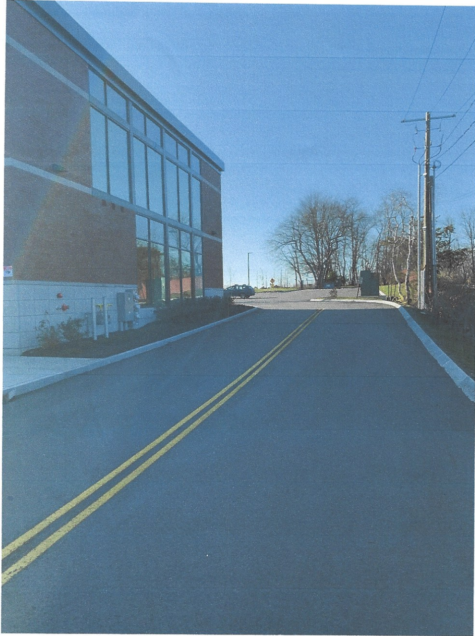
Alternate View of Building from Cottage Street (South)
