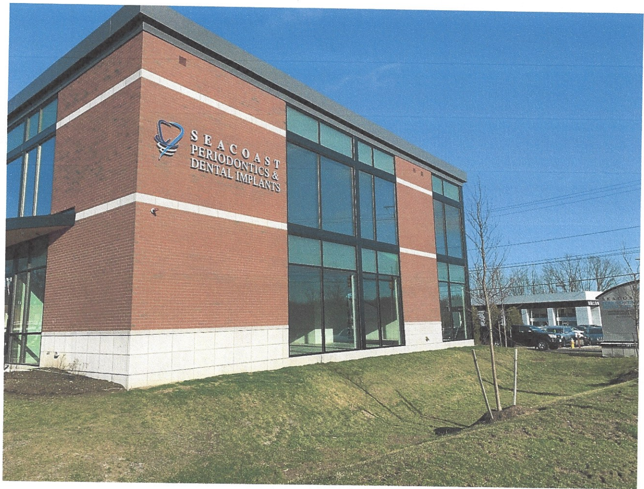
View of Building From Lafayette Road (West)
