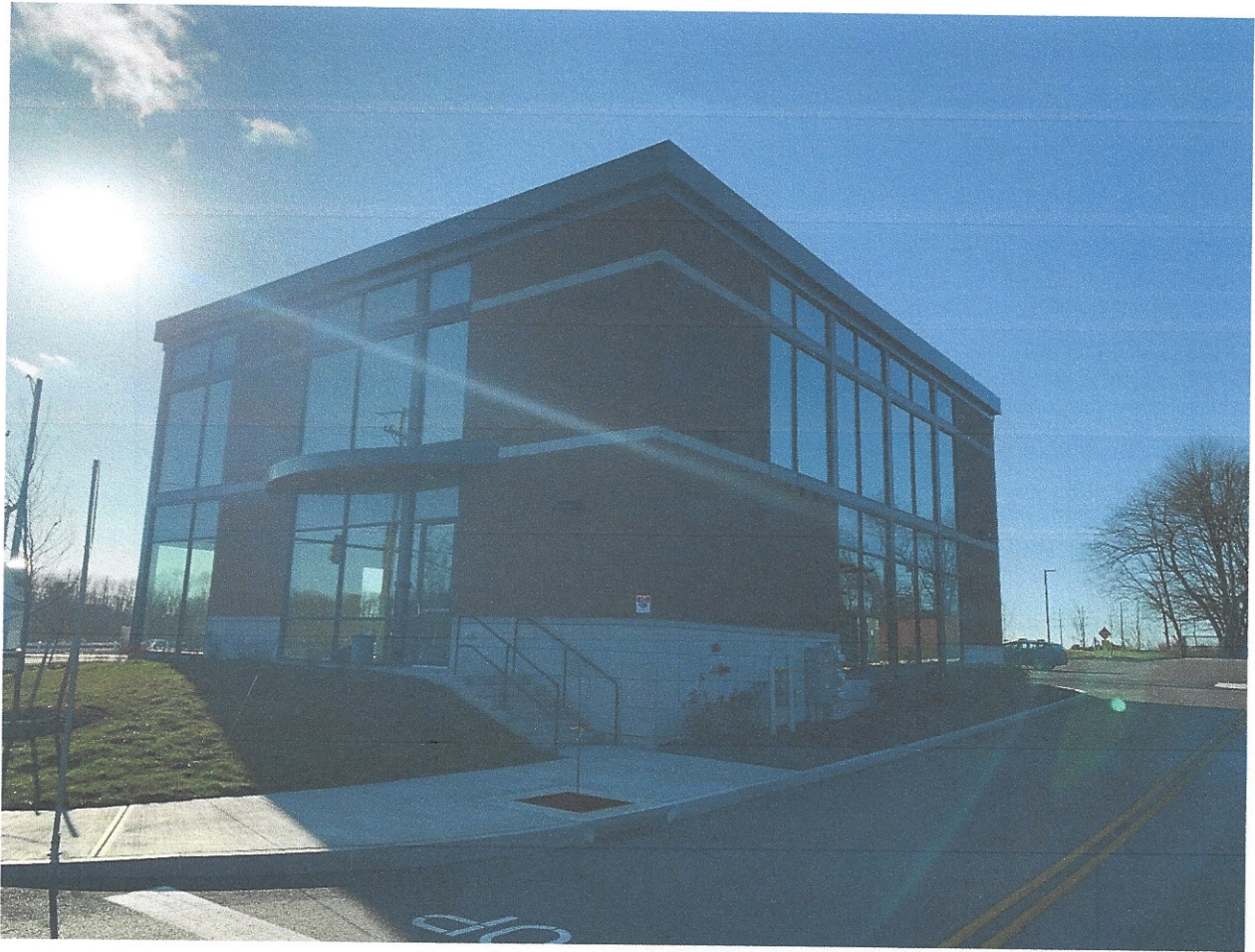
View from Cottage Street / Rear of Building (SouthEast)
