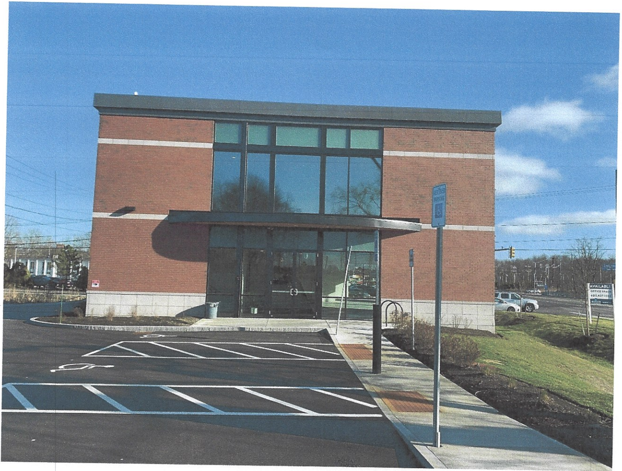
View of Building from Parking Lot (North)
