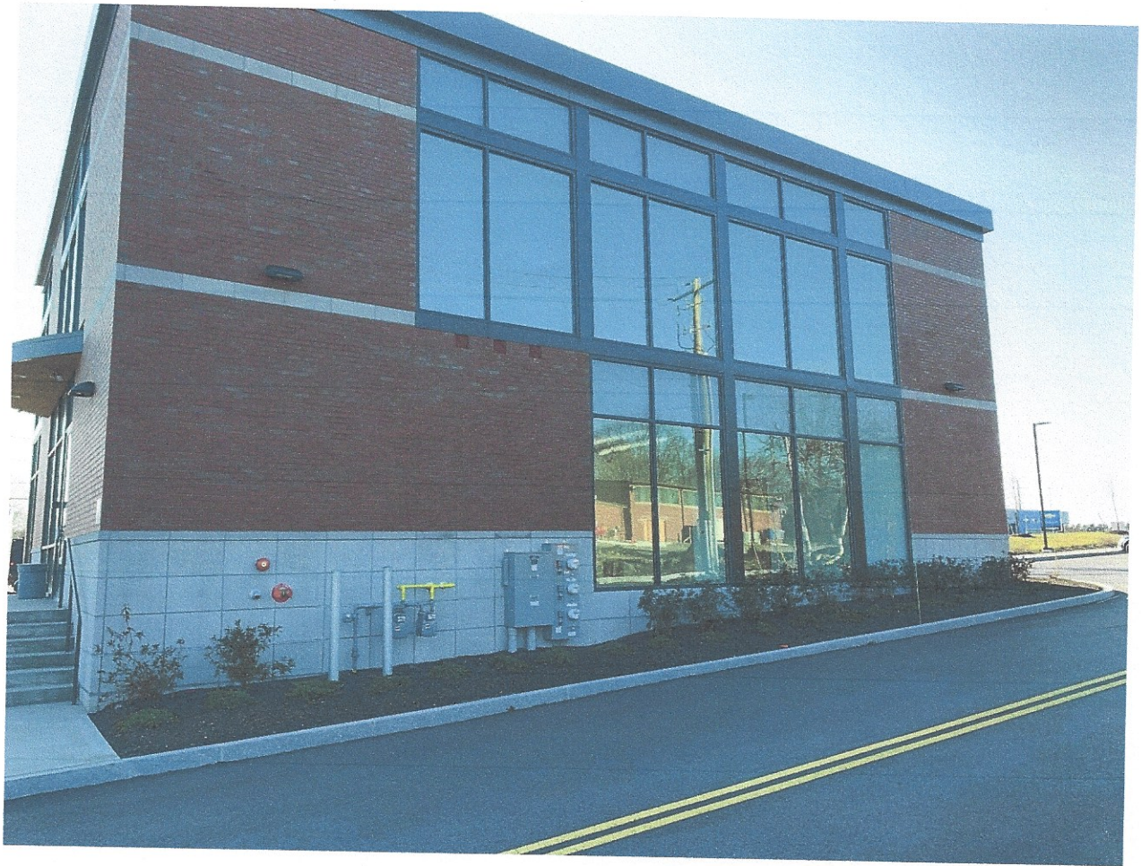
View of Building from Rear / Cottage Street (East)
