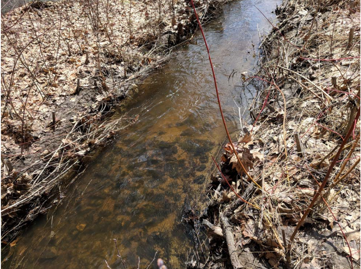
Figure 2 - Coir Log Rolls along Restored Pettee Brook, near Adams Towers on UNH Campus in Durham, four years after construction. Note how the coir logs are still intact, and have trapped sediment. Roots and grasses have grown into and through them.
