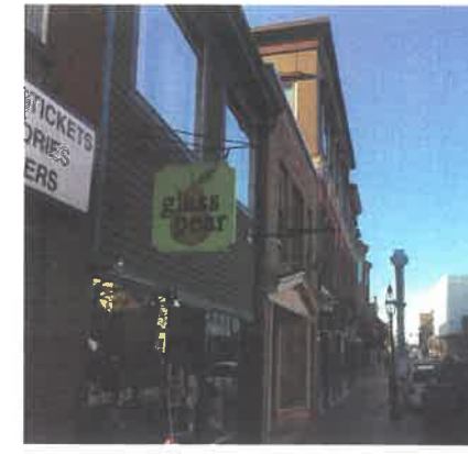
6 - 2018 view down Congress St. w/ recent modifications in context
