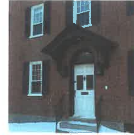
3 - open pediment over Atkinson St. doorway
