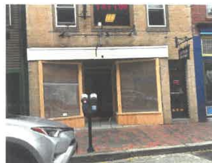
2 - 2018 facade w/ vertical panels below new storefront windows & previous sign board above
