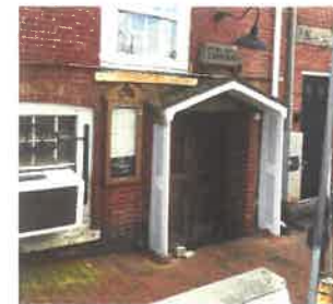
2 - open pediment over Ceres St. doorway
