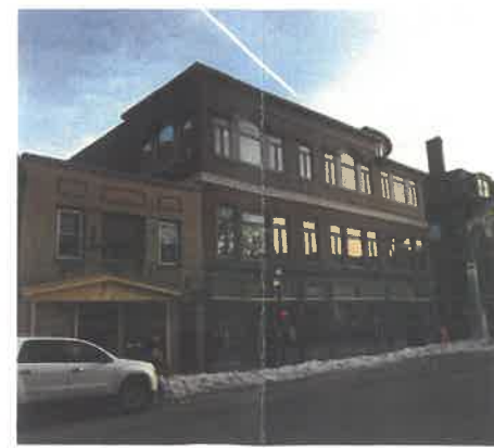
5 - 2018 view down Congress St. w/ facade modifications
