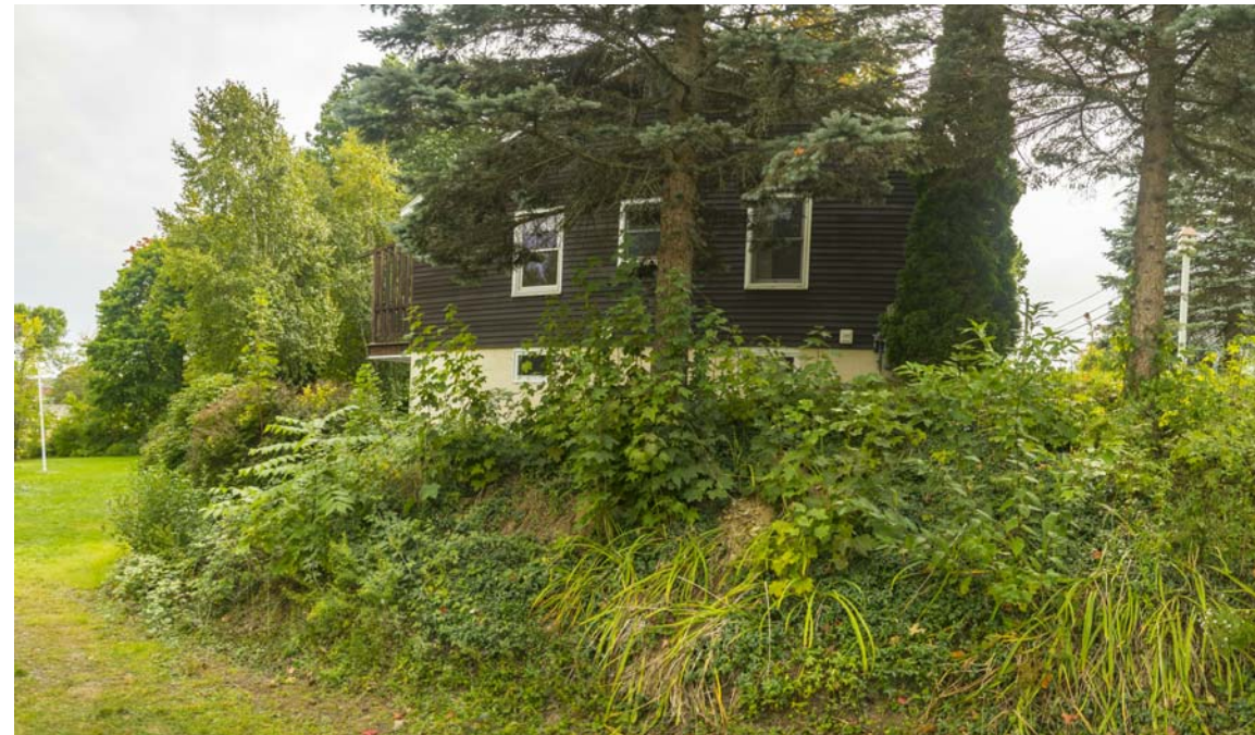
VIEW FROM LEFT SIDE YARD
