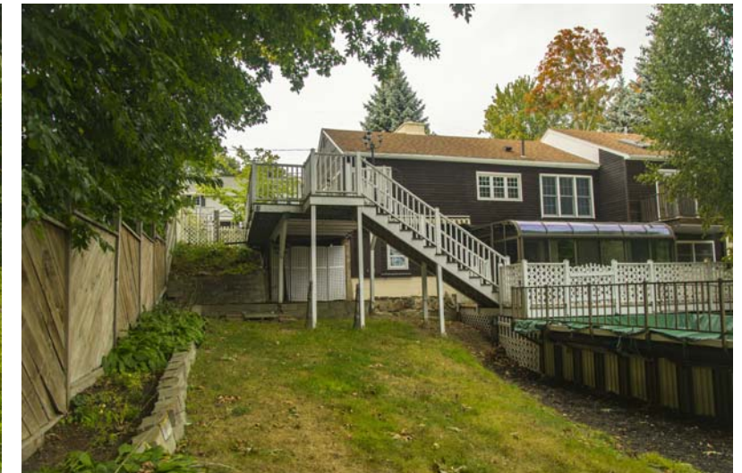
VIEW FROM REAR AT PROPERTY LINE
