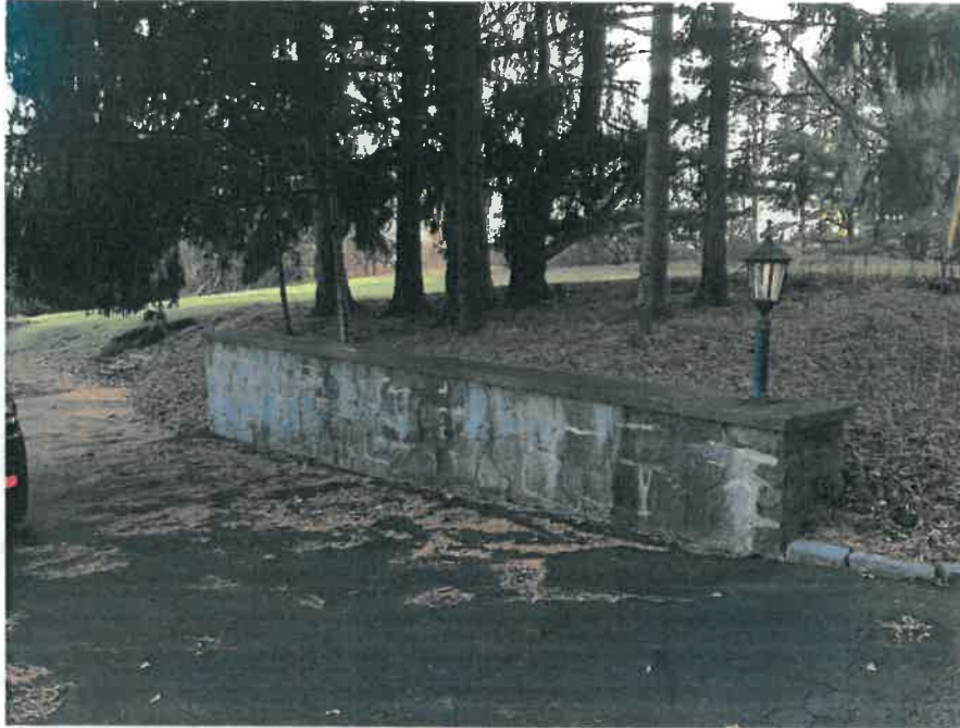
Photo #5: Looking southerly at existing retaining wall to be removed. November 24, 2020
