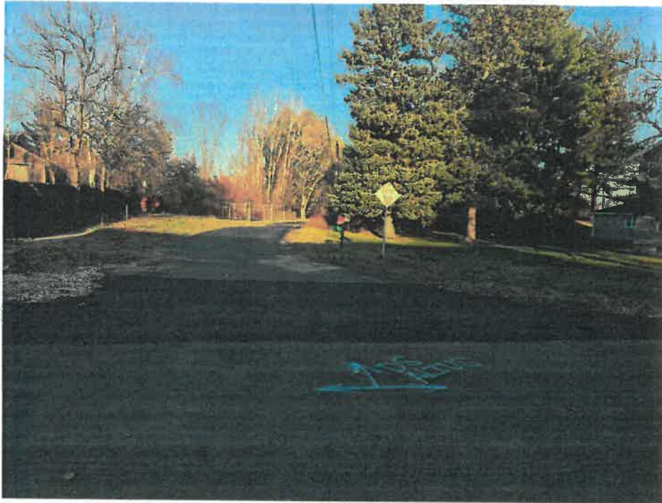
Photo #1: Looking northeasterly at existing driveway to be replaced with paved cul-de-sac for accessing new lots. – November 24, 2020
