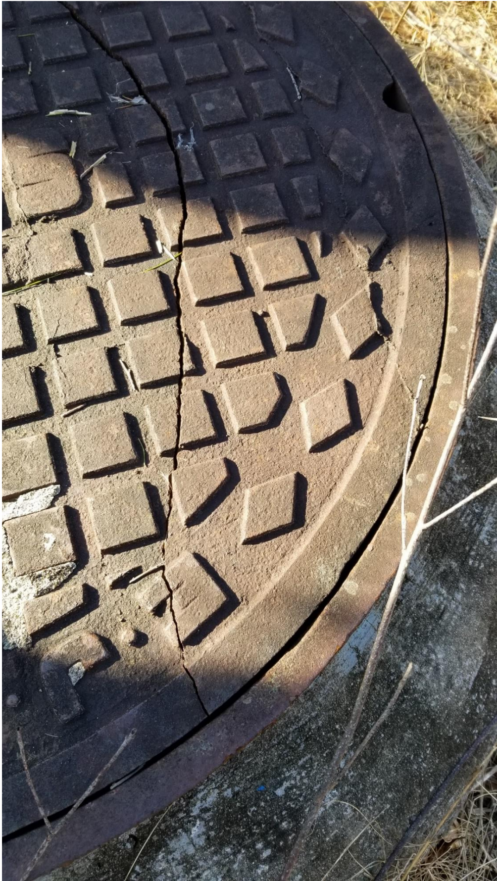
PHOTO V SMH #2458, CRACKED COVER
