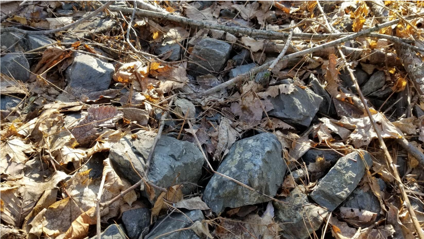
PHOTO C EXISTING STONE BASE IN SEWER EASEMENT
