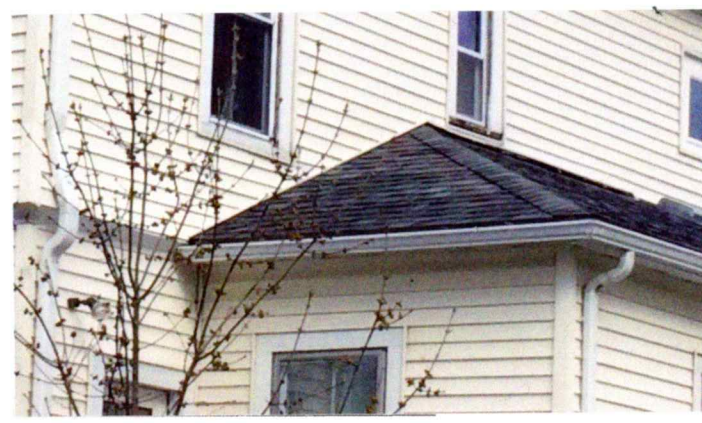
VIEW OF REAR 1-STORY HIP ROOF
