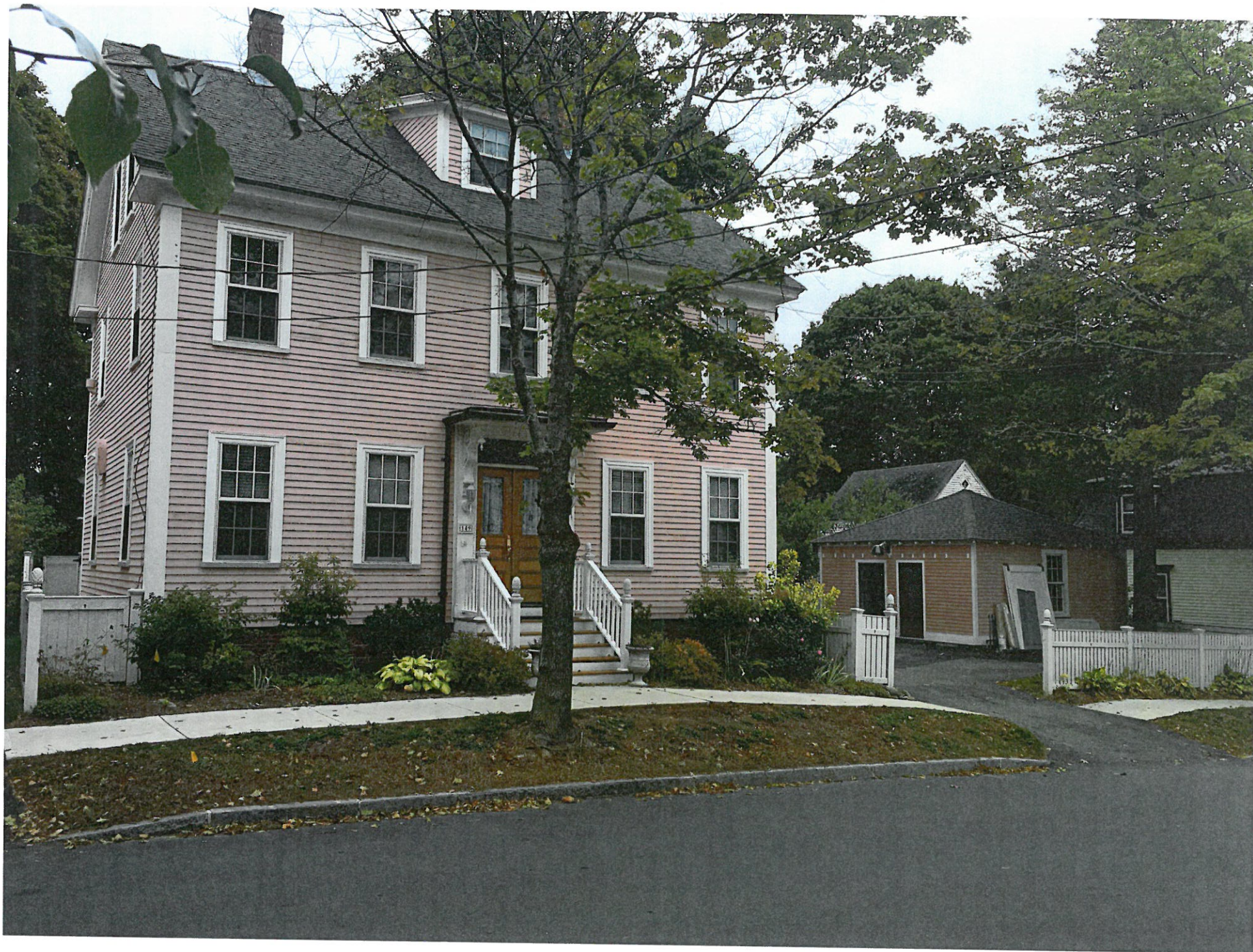
FROM CASS ST FACING EAST
