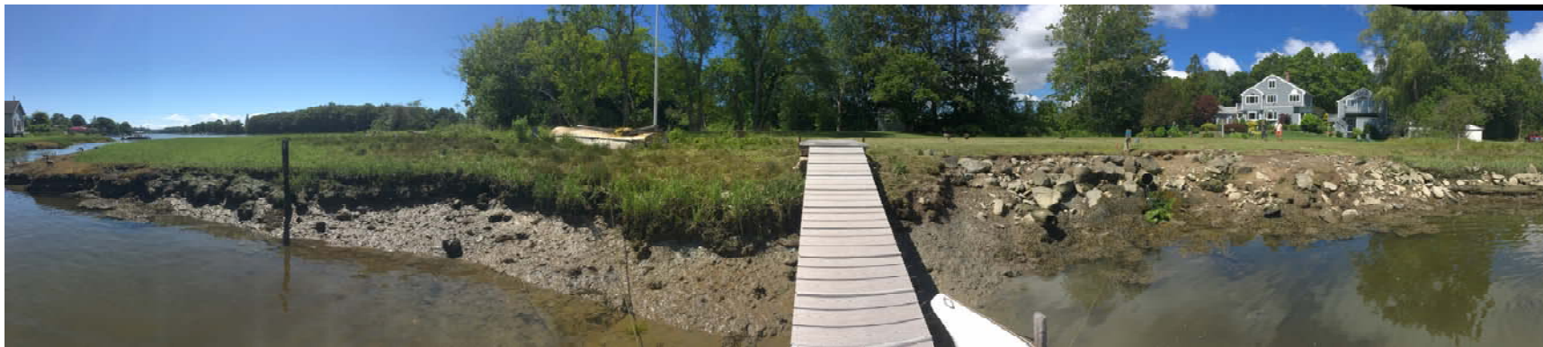
Photo #12: Looking southerly from end of dock at eroded stone areas. Embedded stone will be replaced and strengthened in this area. July 15, 2020
