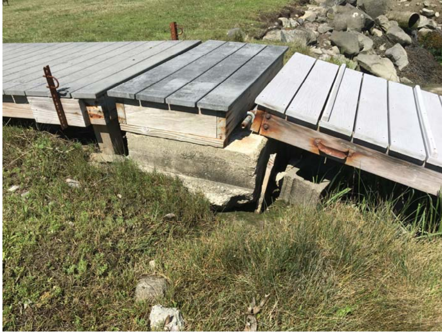
Photo #3: Looking northwesterly at concrete dock support to be replaced. July 15, 2020
