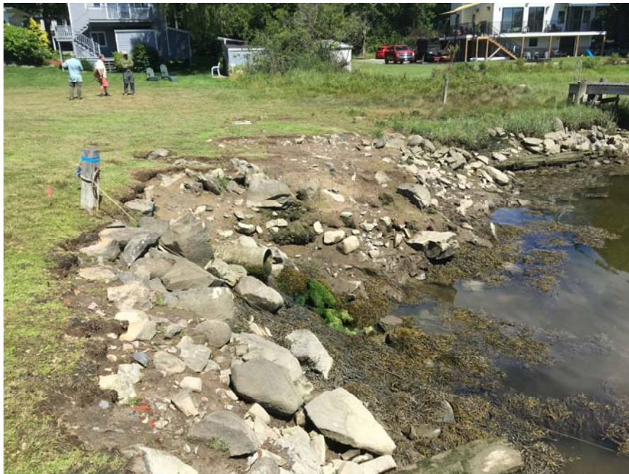
Photo #4: Looking northwesterly toward drainage pipe outfall and eroded embedded stone slope. Proposed raingarden outfall to be located in same area and stone areas repaired or replaced. July 15, 2020
