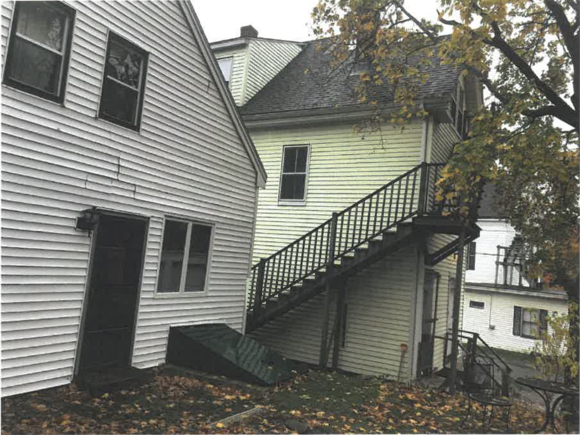
Here you can see the proximity of the house to the abutting structure to the south. The house was built facing south and so the original front door opens only a few feet from the nextdoor building.
