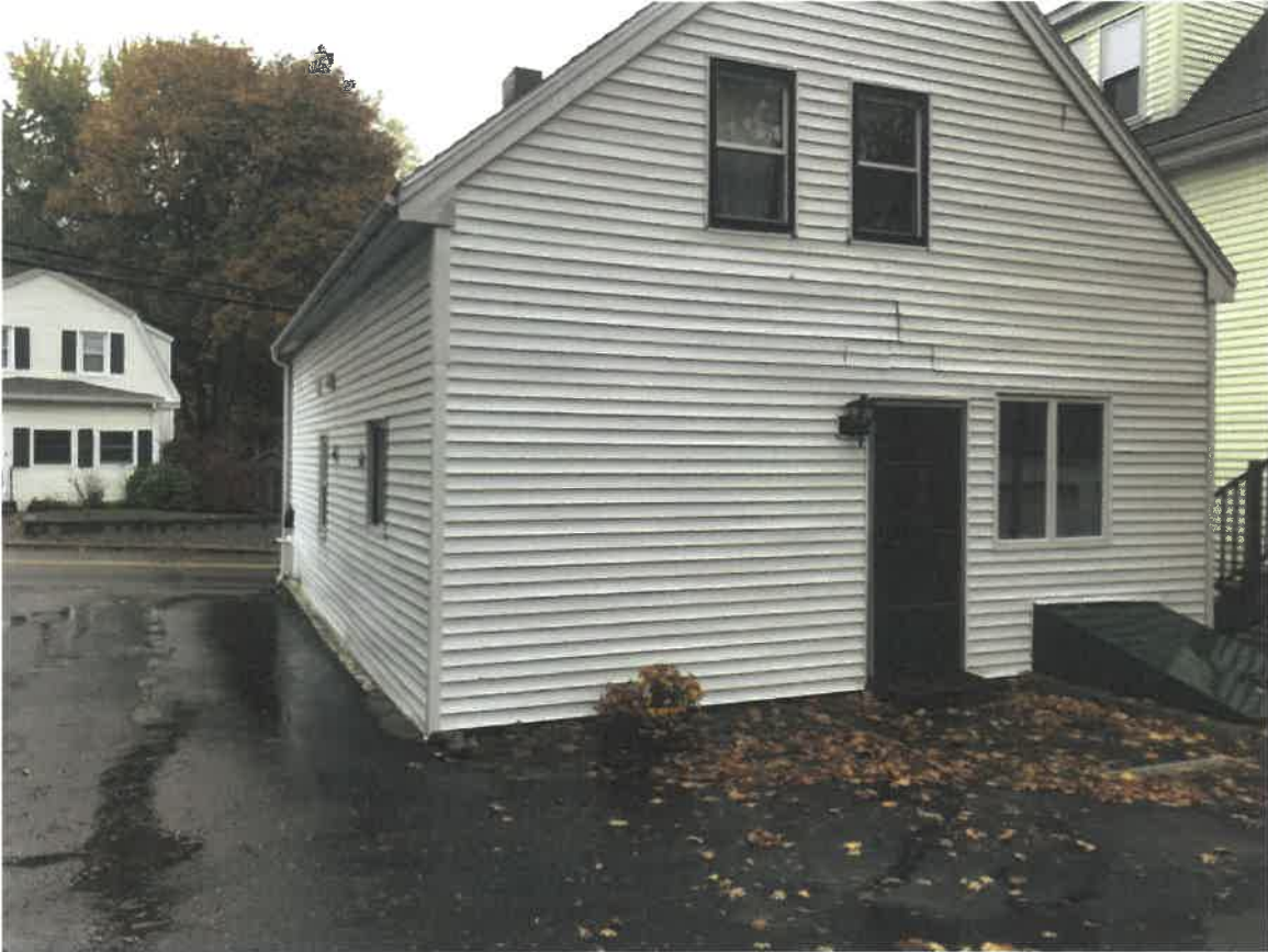
Labeled photo(s) of existing conditions
