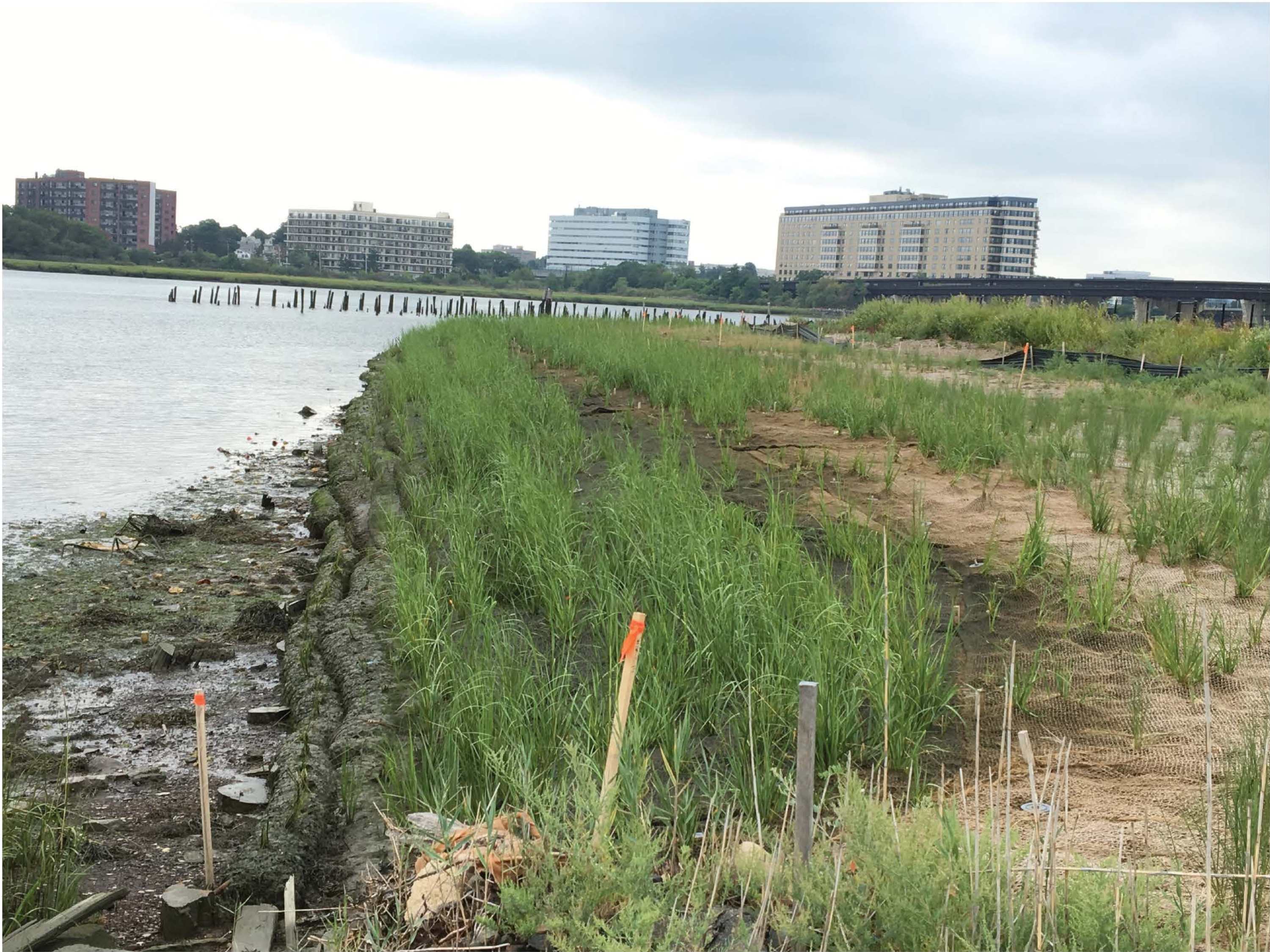
COIR LOGS & STRUCTURAL GEOTEXTILES
