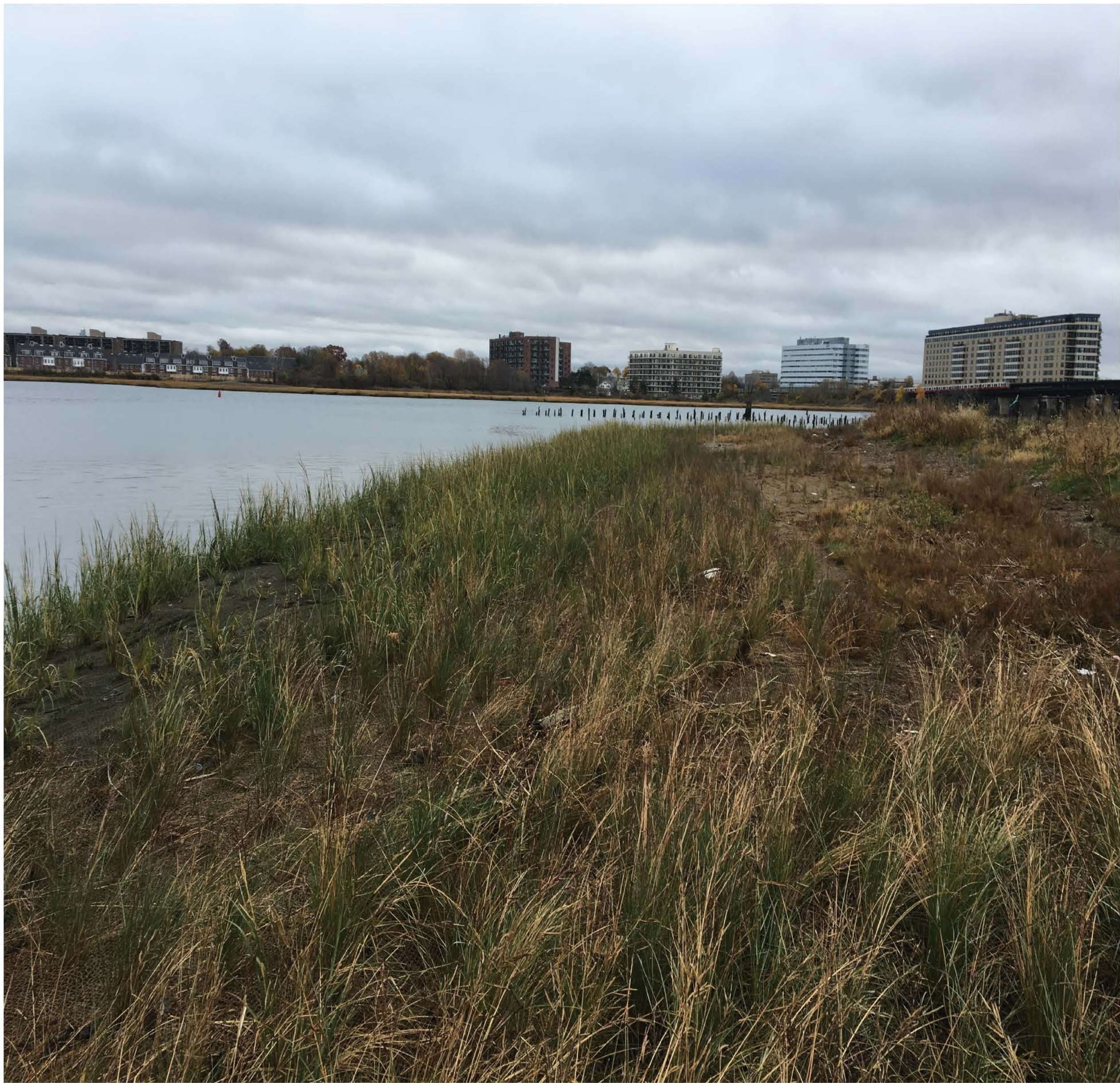
COIR LOGS AND HIGH AND LOW MARSH PLANTINGS AFTER TWO YEARS OF ESTABLISHMENT
