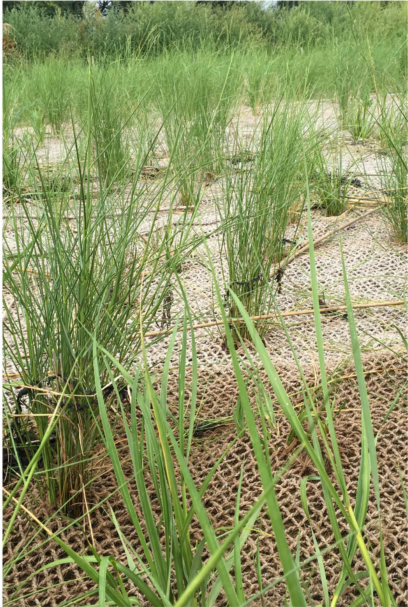
MARSH GRASS PLANTINGS INSTALLED WITH COIR BLANKET
