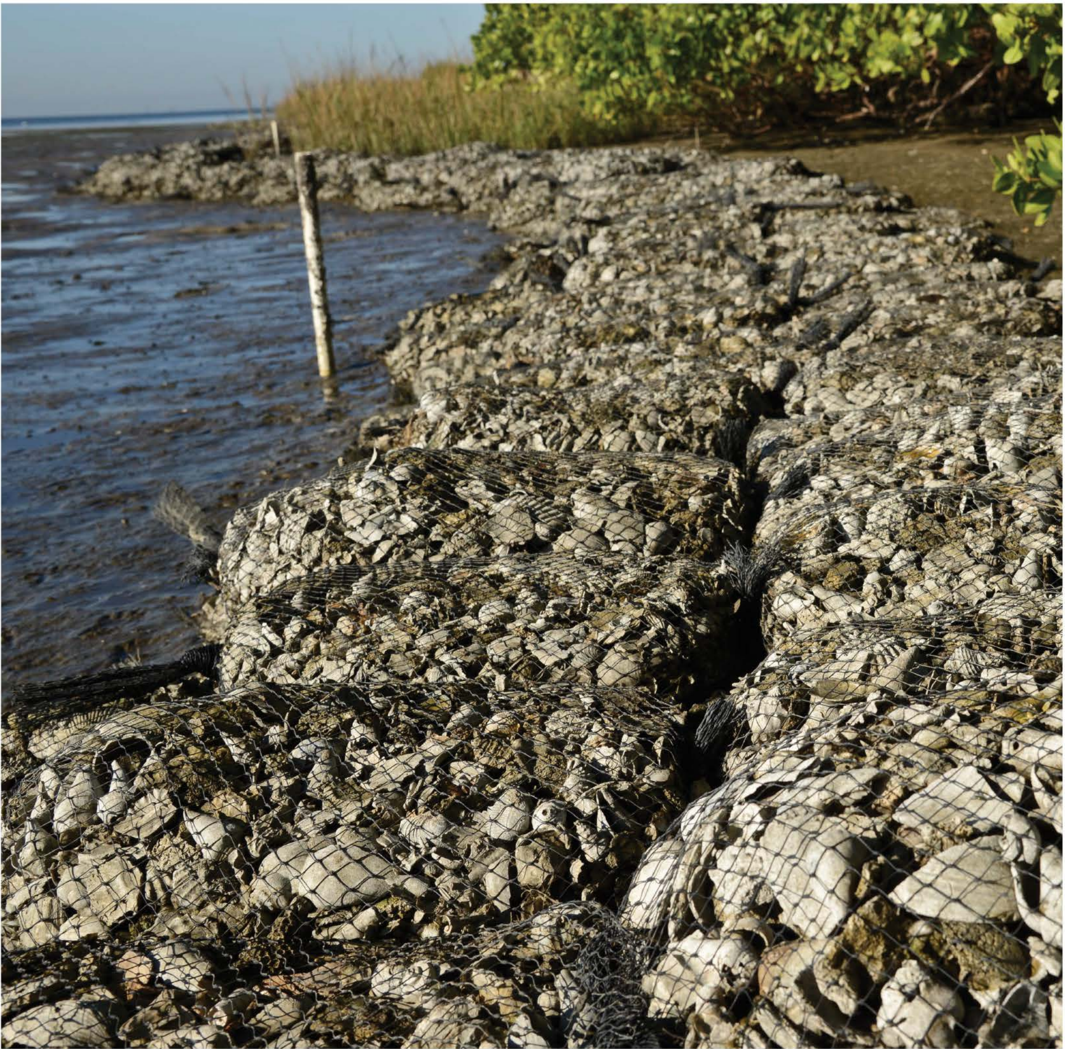
GABIONS WITH OYSTER SHELL AND ROCK
