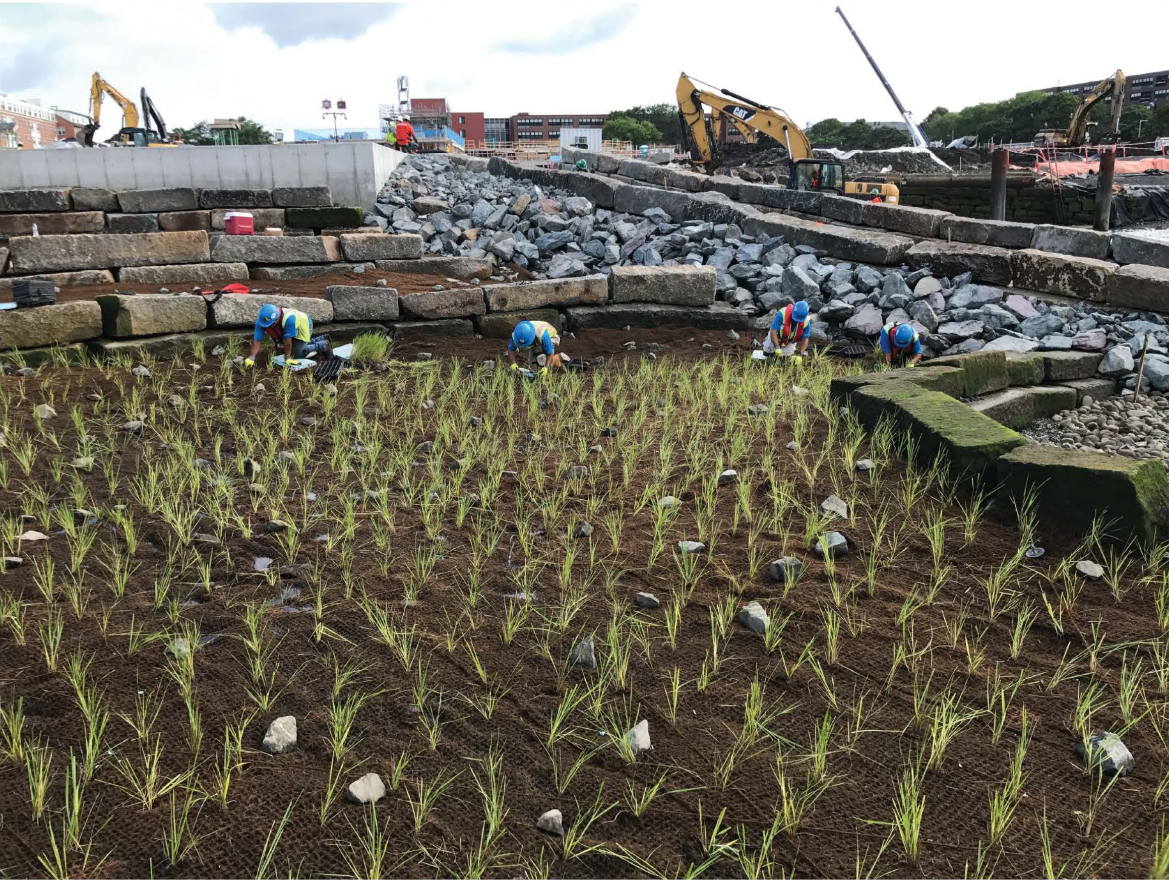
SALVAGED GRANITE BLOCK CELLS
