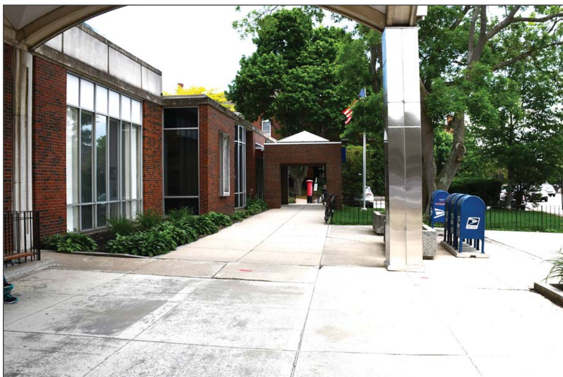
4. South elevation, facing east
