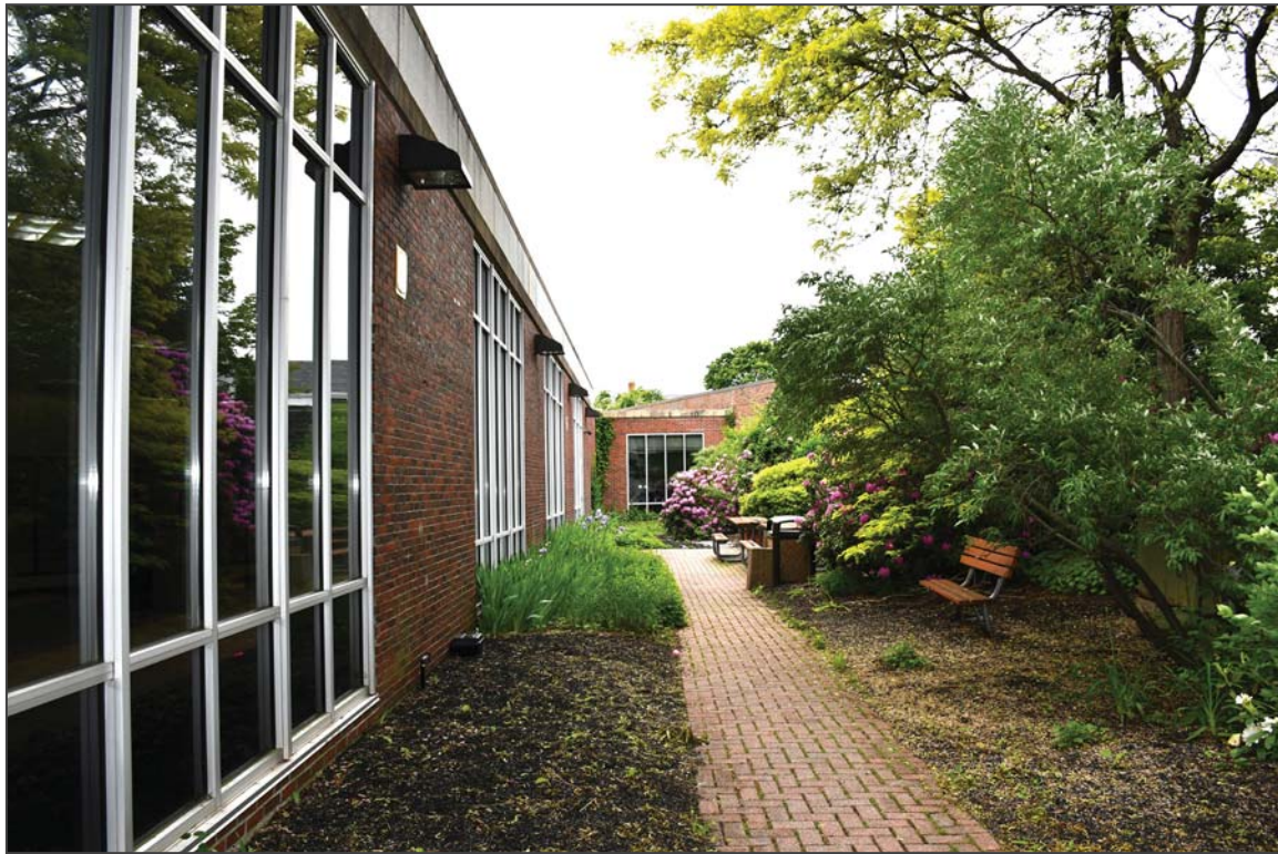
11. East and south elevations, facing north
