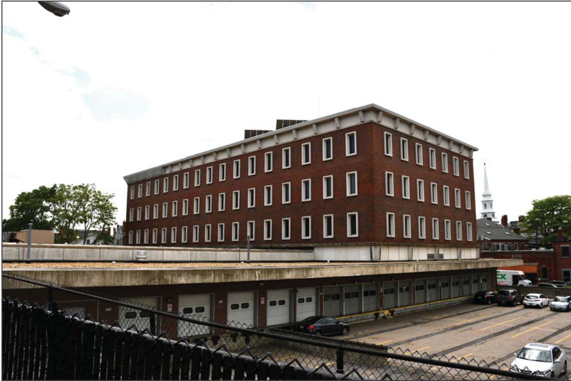
13. East and north elevations, facing southwest
