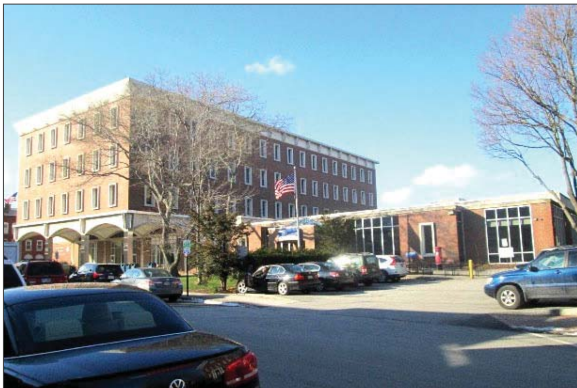
9. South and east elevations, facing northwest
