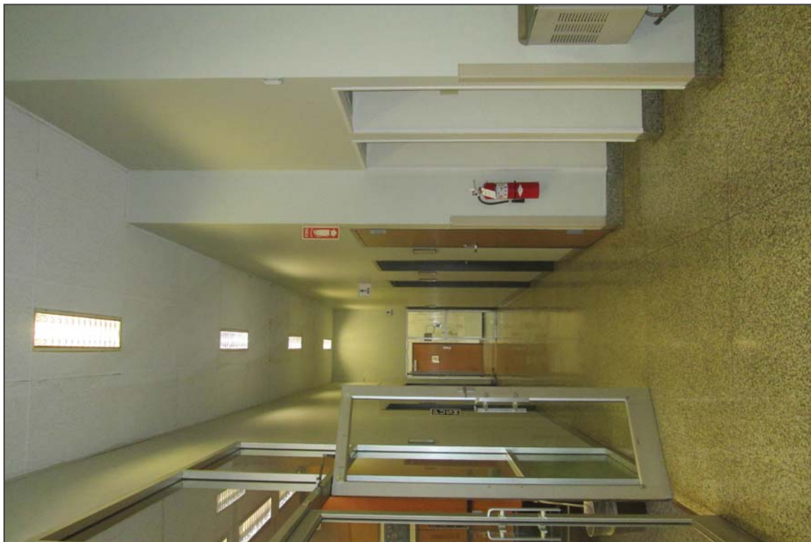
48. Ground floor, facing north
