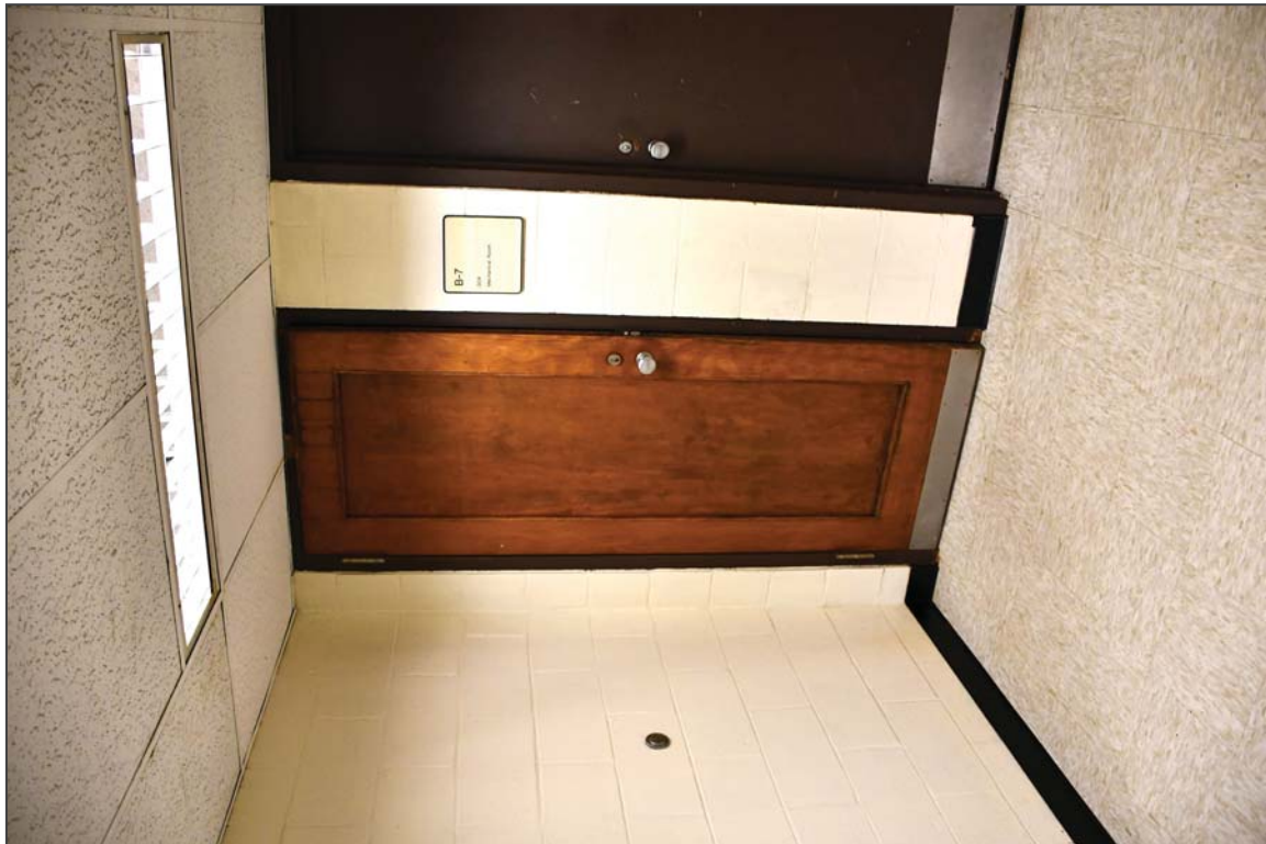
29. Basement, facing west
