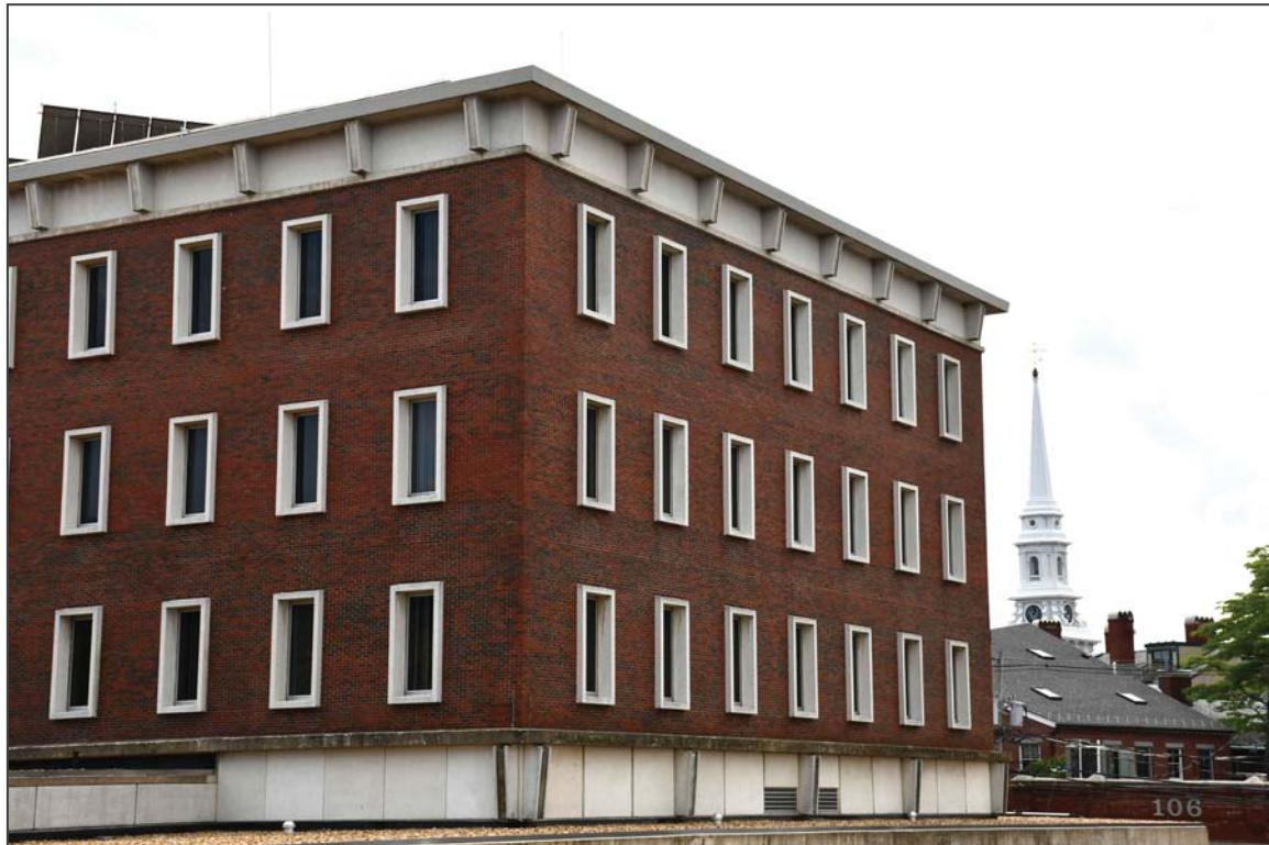
15. East and north elevations, facing southwest
