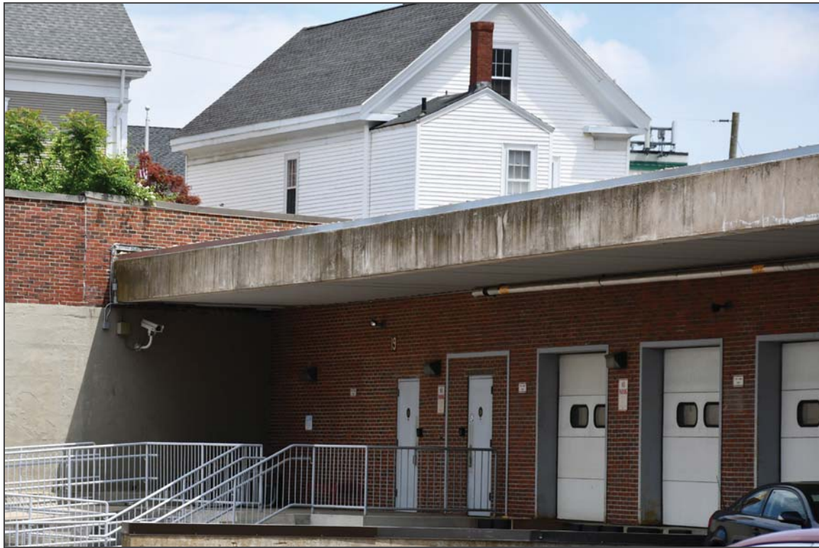
19. North elevation, facing southeast
