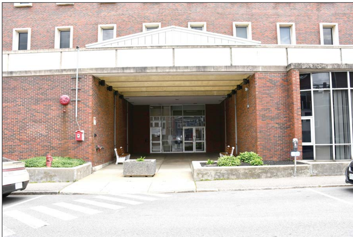
23. West elevation, facing east
