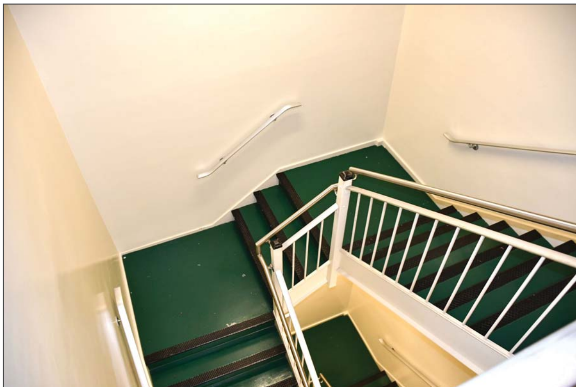
65. Fourth floor, facing southwest
