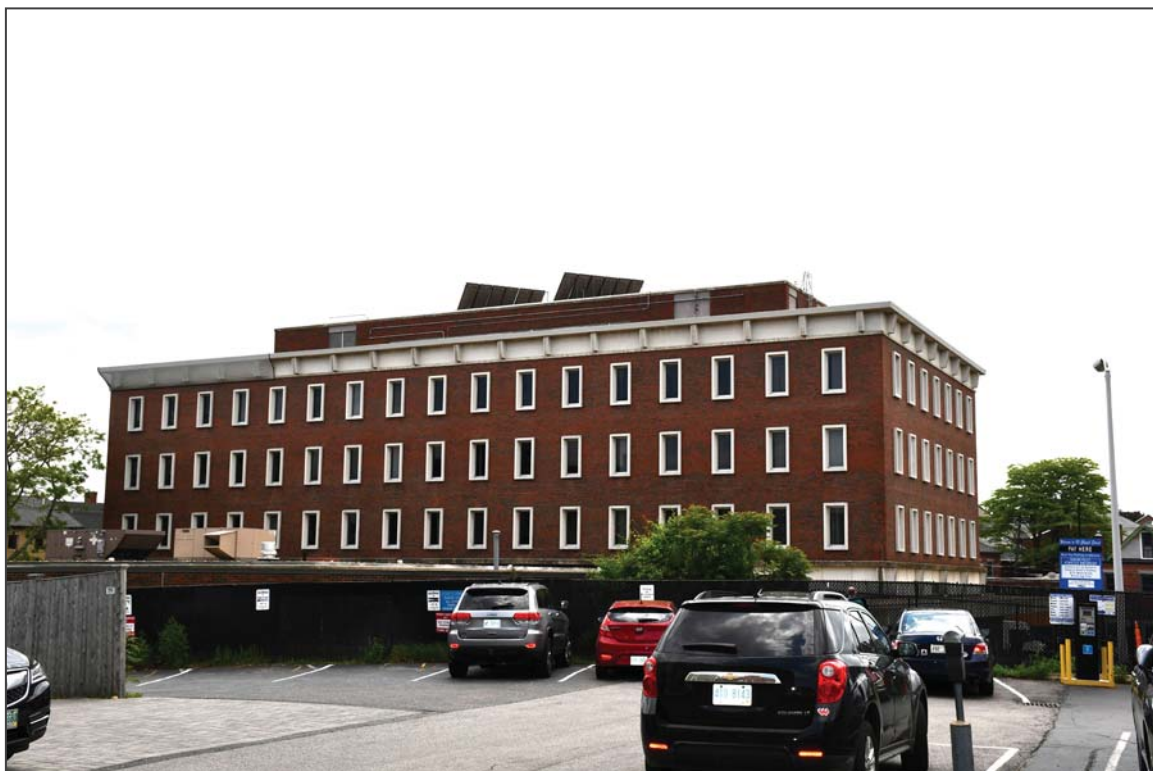
12. East and north elevations, facing southwest
