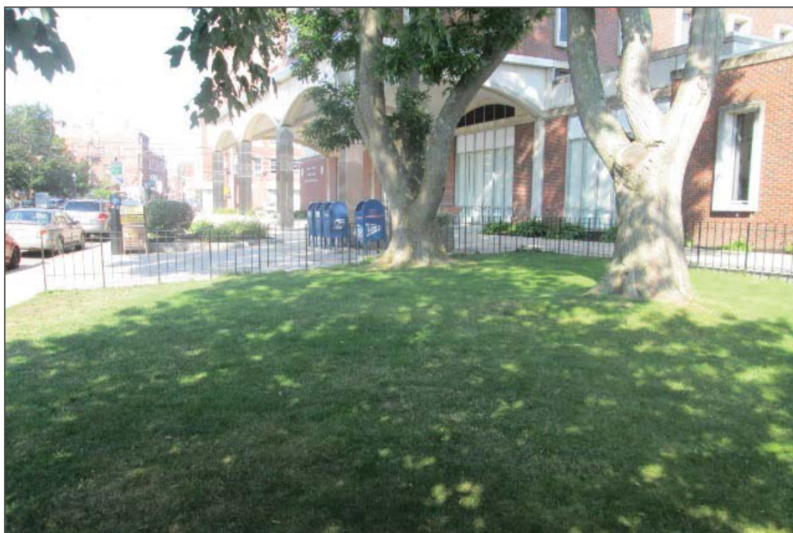
10. Site and south elevation, facing northwest
