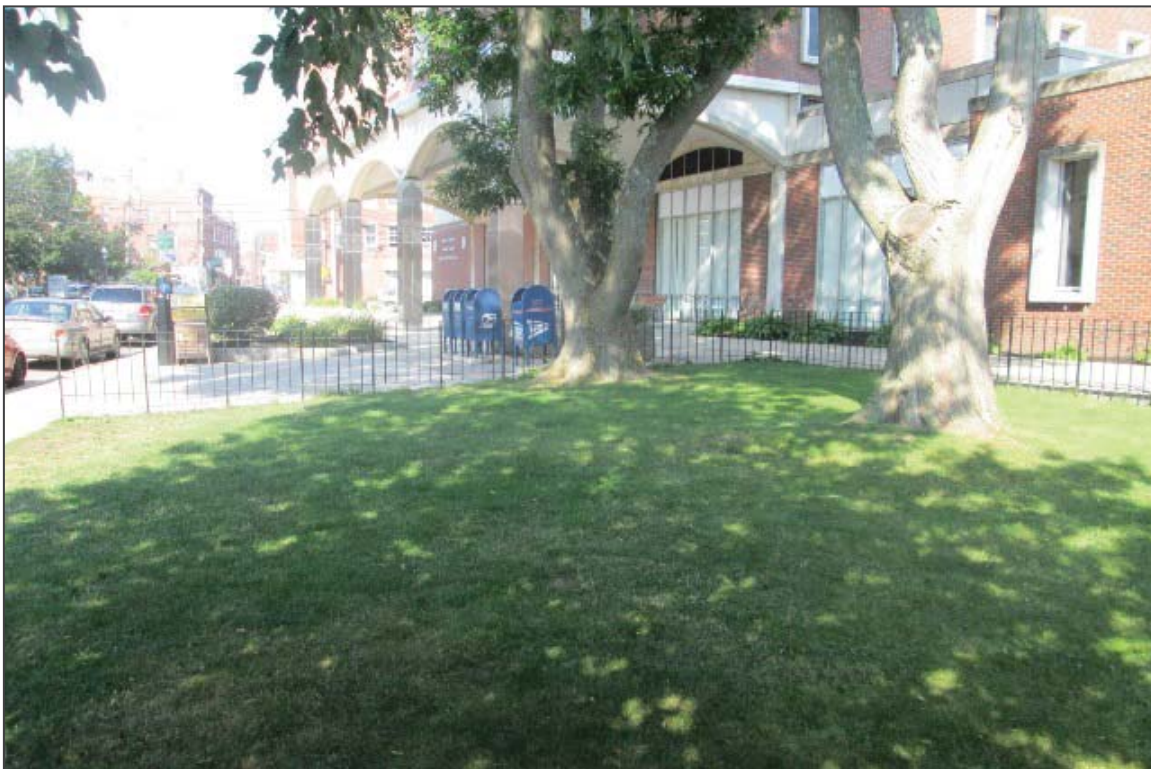
10. Site and south elevation, facing northwest
