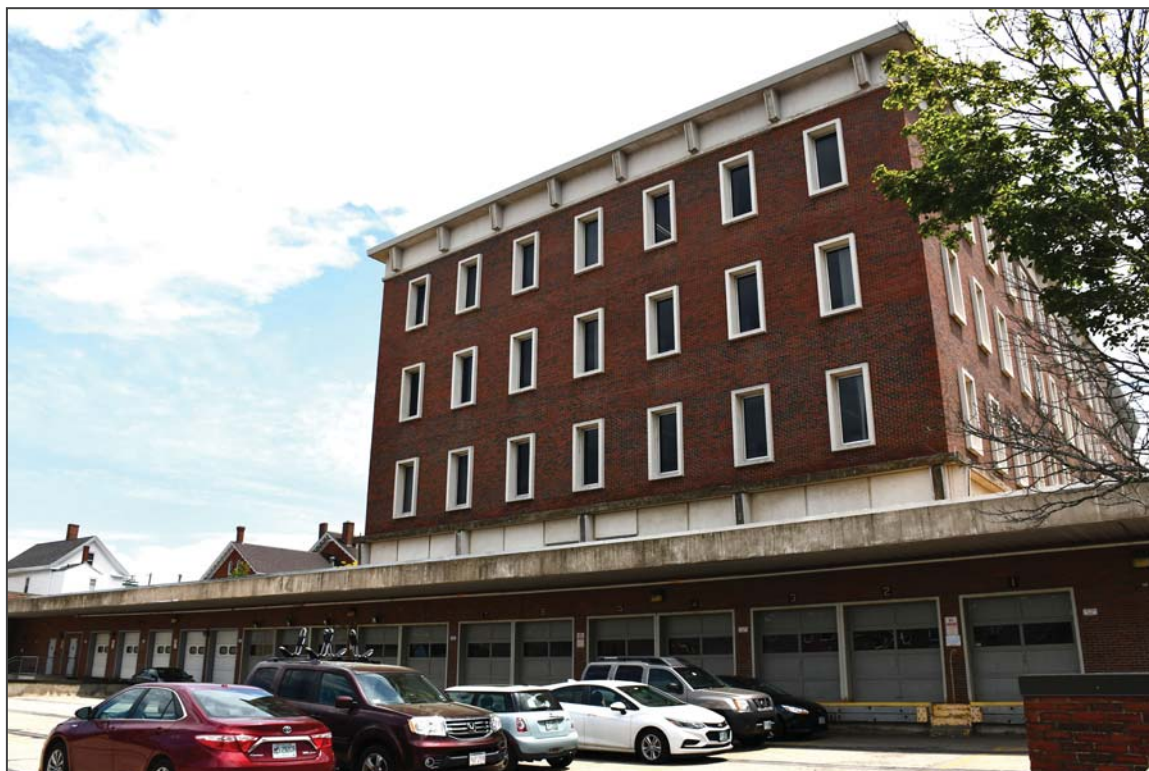
17. North elevation, facing southeast
