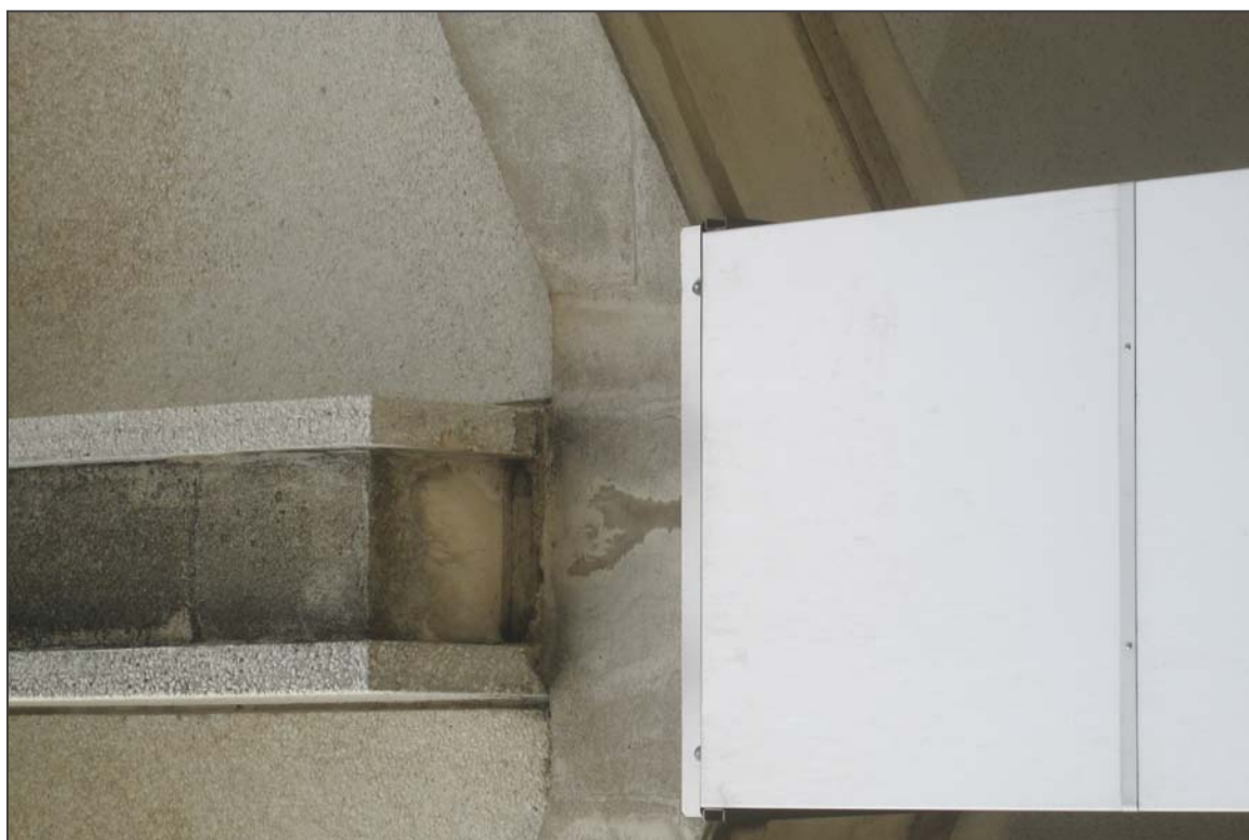
28. South elevation column detail
