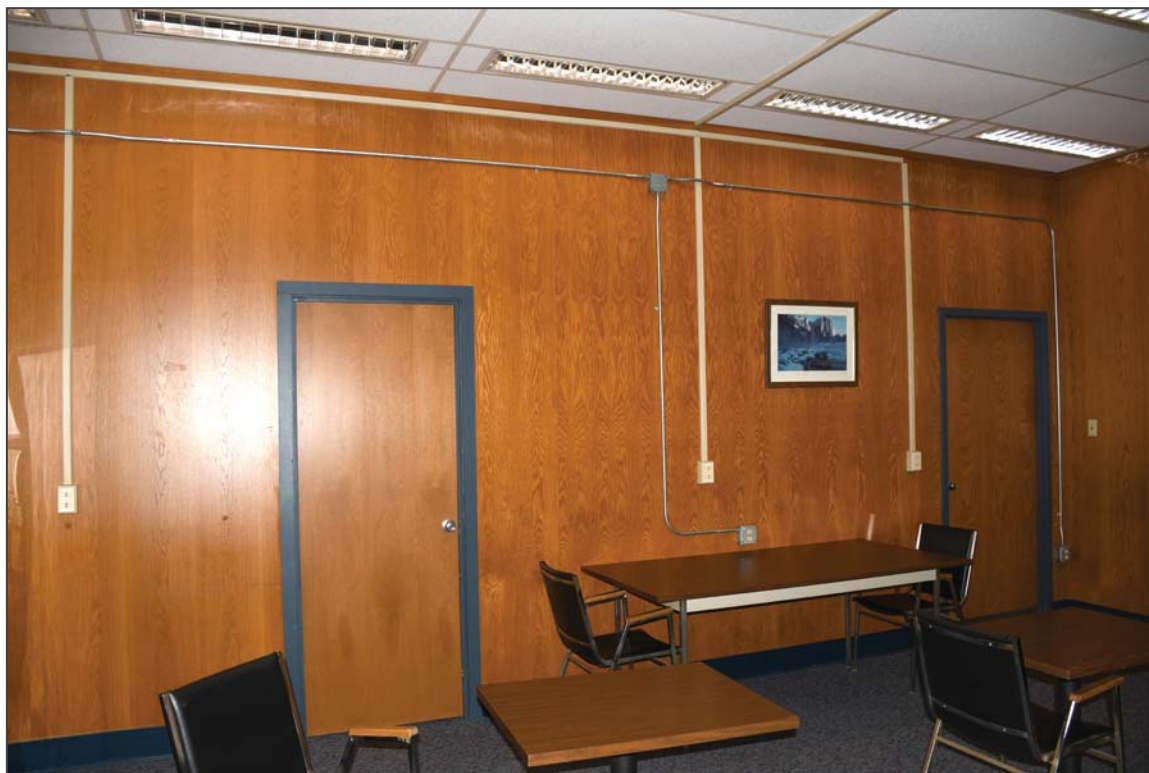
47. Ground floor, facing northwest
