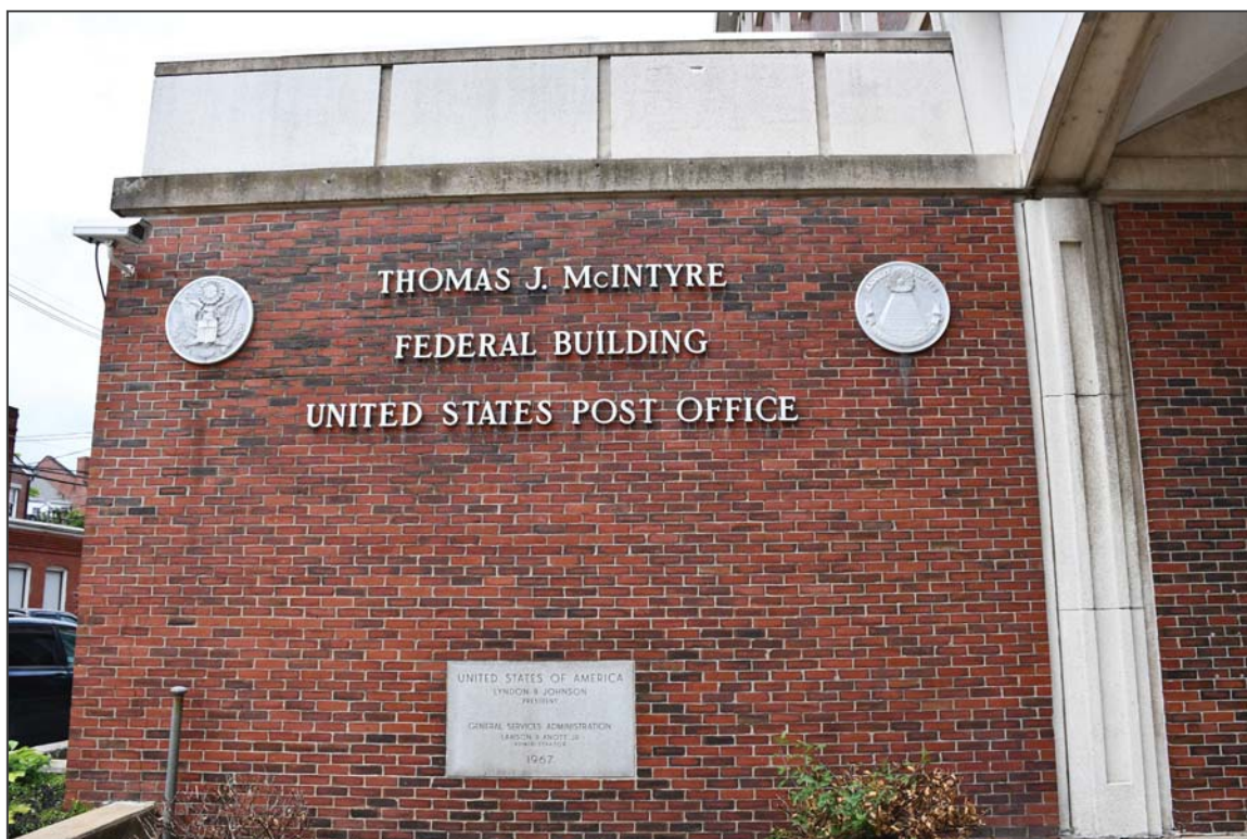
2. South elevation, facing north
