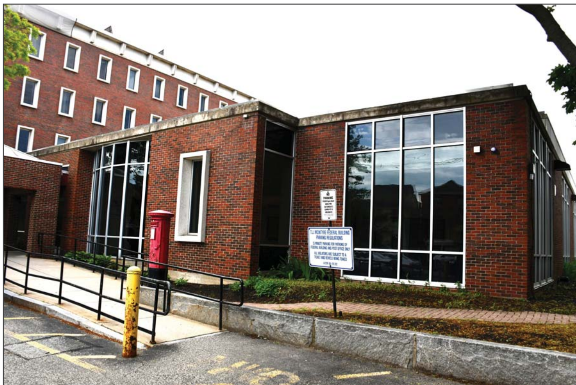
8. East and south elevations, facing northwest
