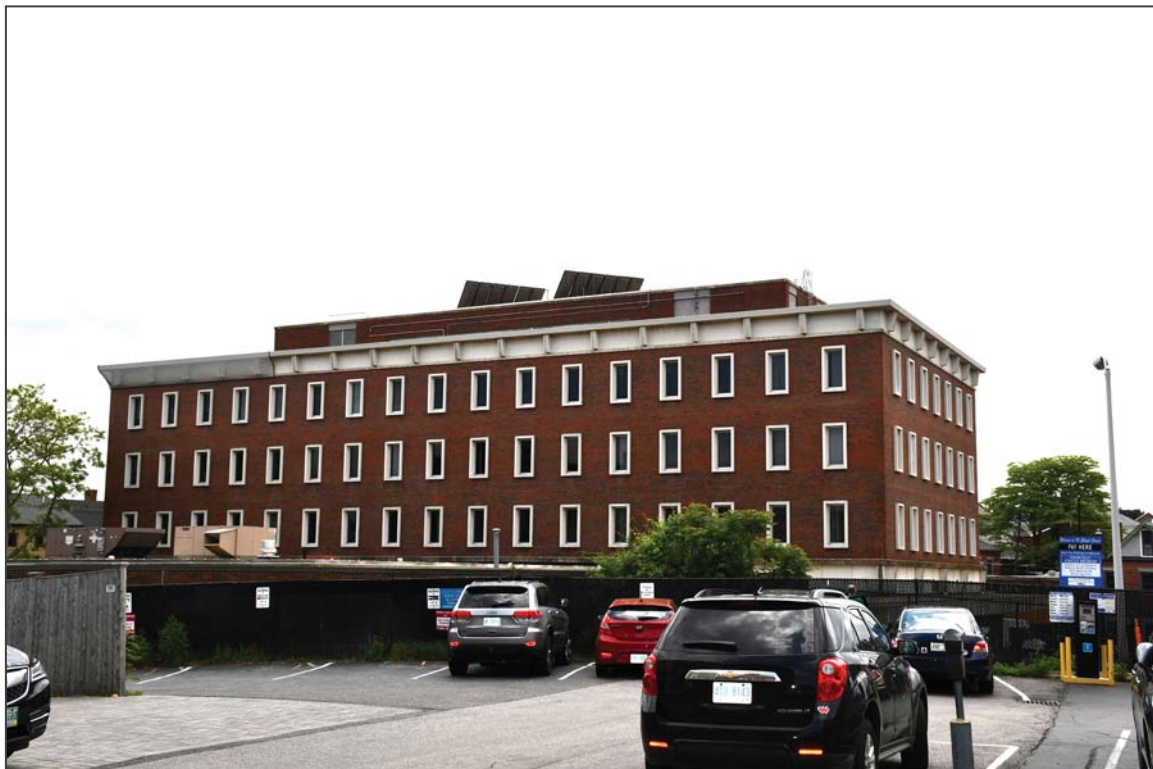
12. East and north elevations, facing southwest
