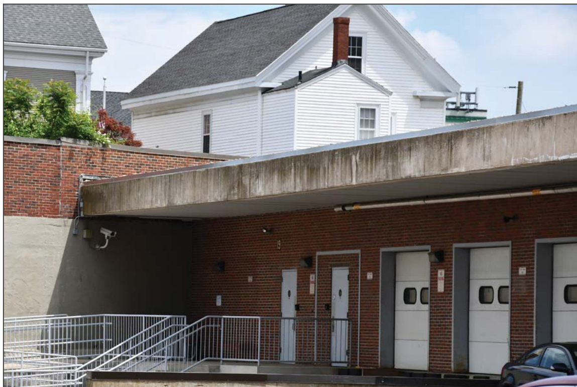
19. North elevation, facing southeast
