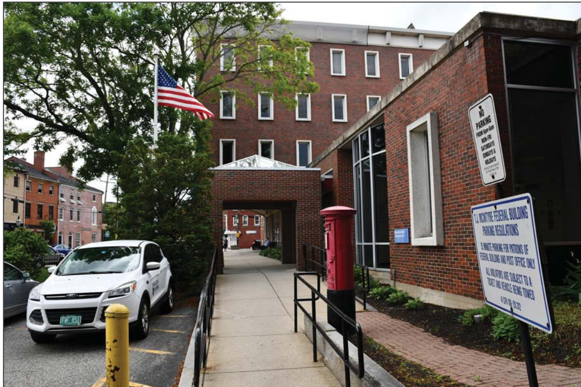
7. East and south elevations, facing west
