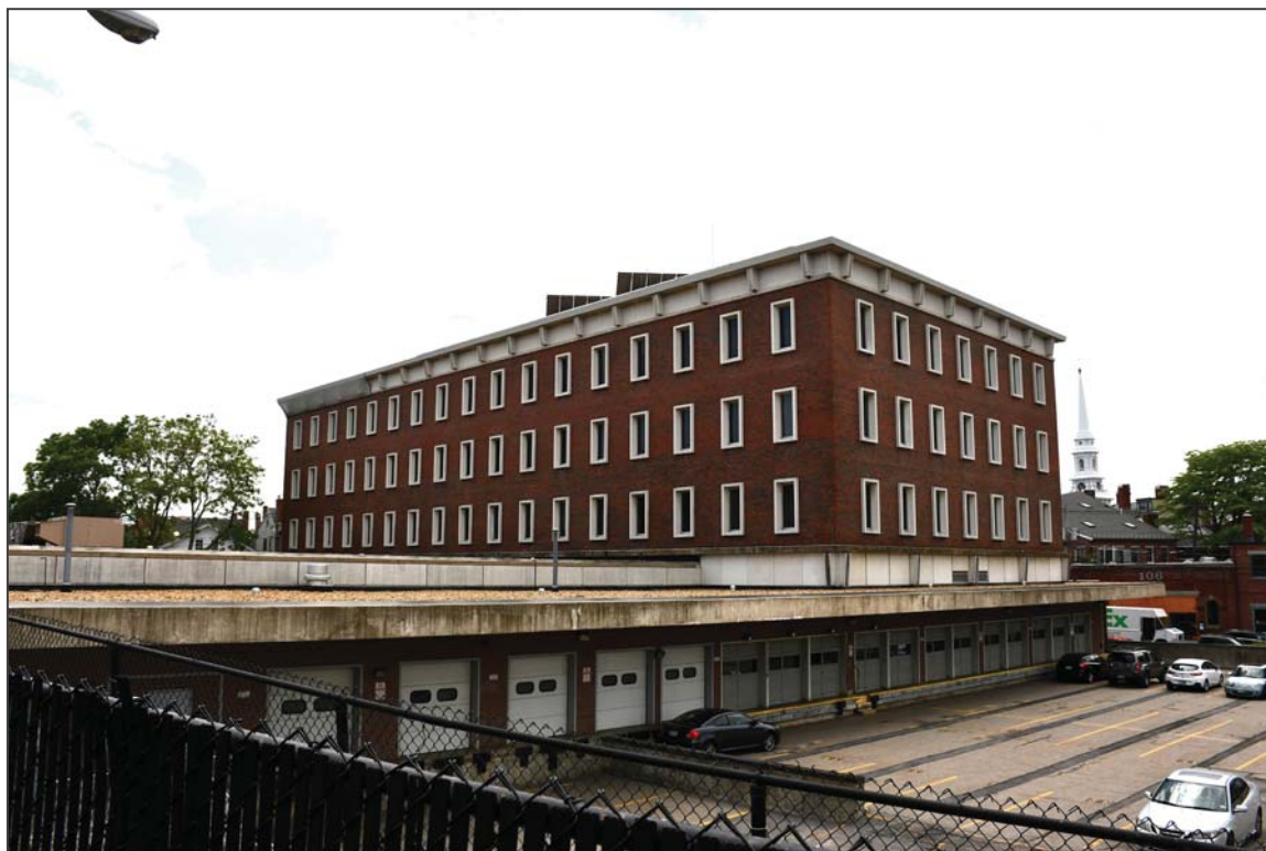
13. East and north elevations, facing southwest
