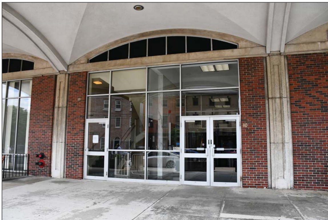
3. South elevation, facing north
