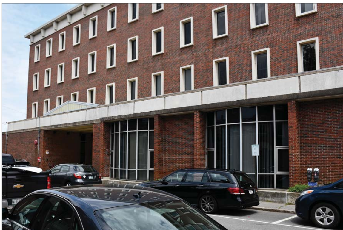
26. West elevation, facing northeast
