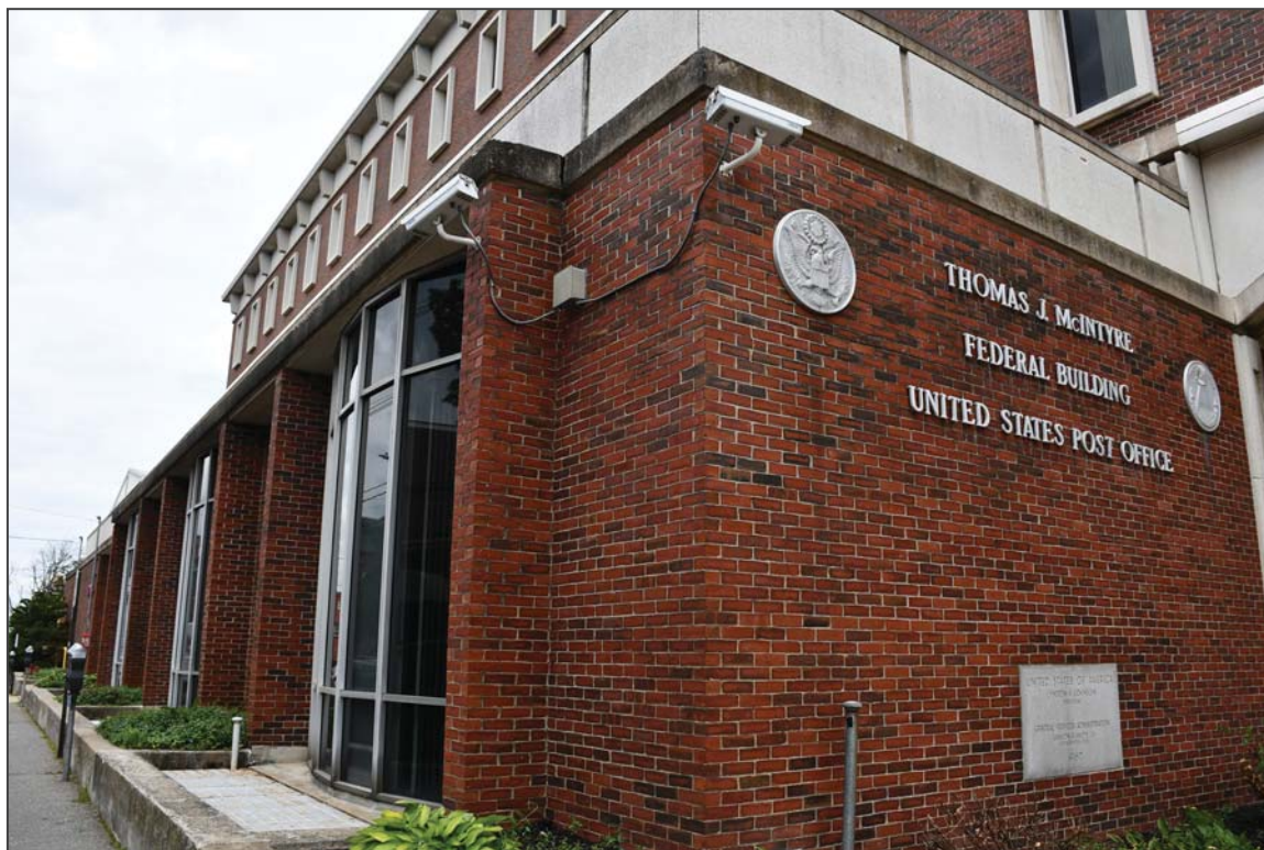
1. West and south elevations, facing northeast
