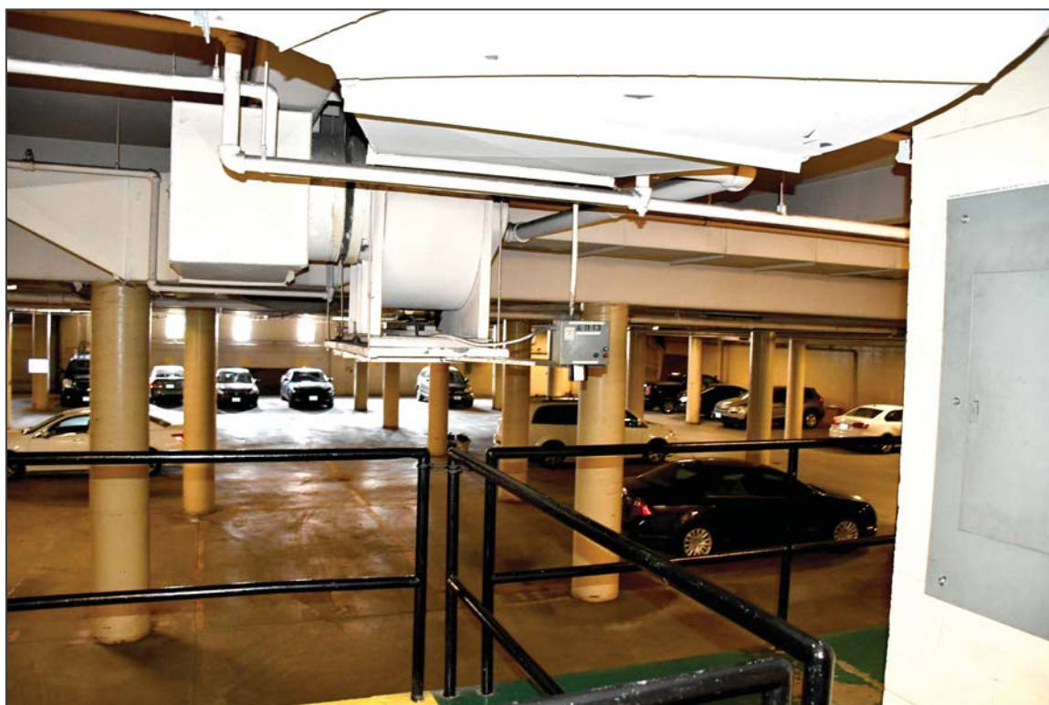
32. Basement, facing northeast
