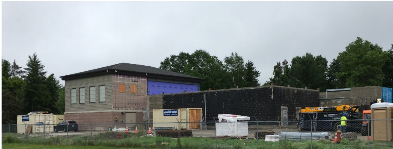
July 2020 Photo of Pease Grafton Road PFAS Water Treatment Facility Construction
