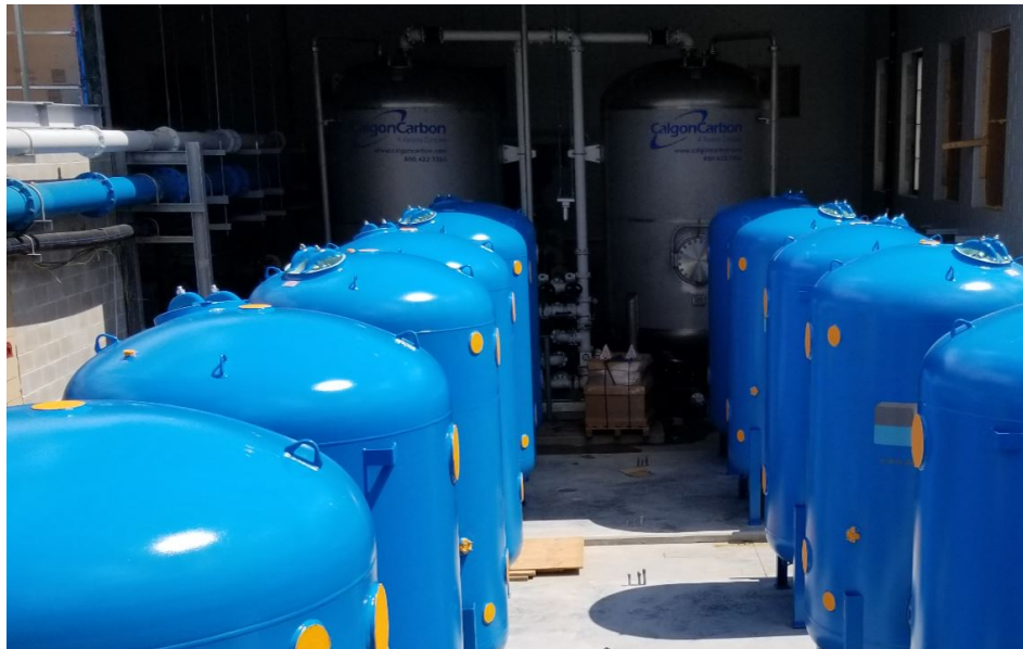
Delivery and Installation of Resin Filter Vessels in August 2020
