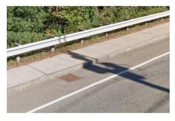
The existing stormwater drainage system is limited to closed drainage systems along the curbed section near Middle Road and from the intersection of Banfield/Mirona Road east to the DPW driveway. Based on an initial field review, the closed drainage structures appear to be in good condition. There are also a number of cross culverts within the project limits that will need to be reviewed as the project moves forward. Several land owners have indicated
