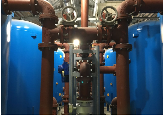
Installation of Piping for Resin Filter Vessels
