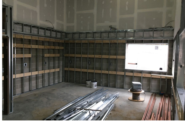
Control Room Construction
