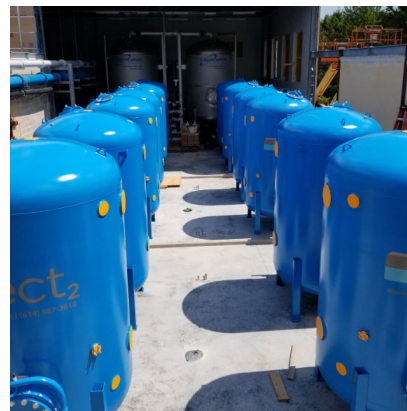
IOX Resin Filter Vessels
