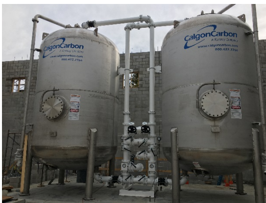
New Granular Activated Carbon (GAC) Filters
