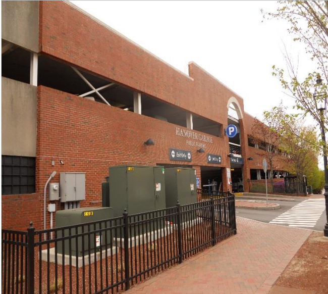
Photo 2 – View of façade northeast corner @ vehicle entry /exit area.
