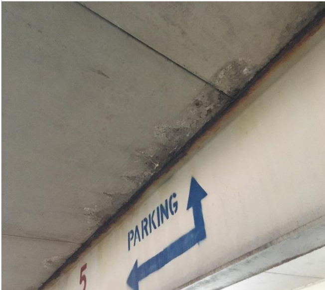
Photo 39 – Floor directional graphics stenciled on steel framing.
