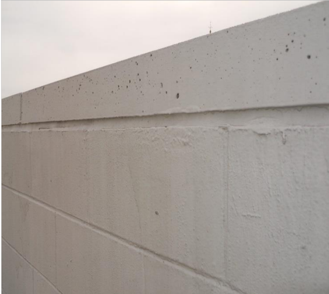
Photo 10 – Waterproofing membrane applied to masonry barrier wall and capstone on level 5.
