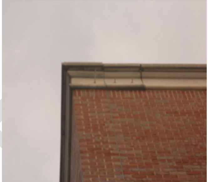
Photo 38 – South façade. Note through bolted connection to secure loose cornice.
