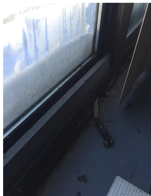
Figure 6: Window with Failed Seals (Typ.)
