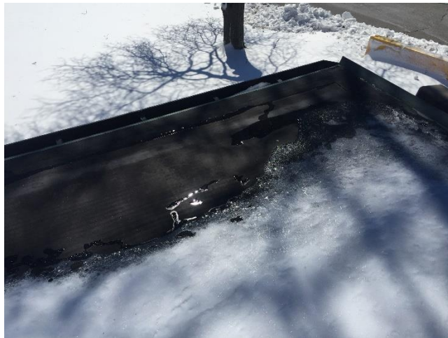
Figure 5: Rubber-Membrane Roofing System
