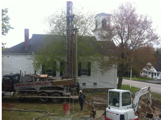
Figure 16: Geothermal Well Construction - Rye Town Hall
