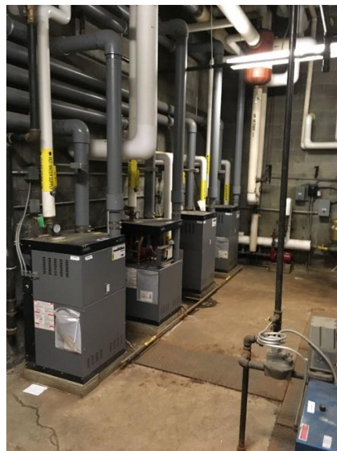
Figure 9: Supplemental Boilers (5)
