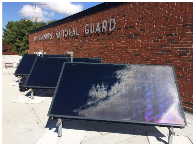
Figure 15: Solar Hot Water Panels - NH Army National Guard, Franklin Readiness Center
