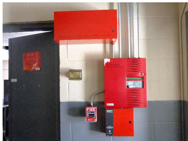
Figure 7: Fire Alarm Panel
