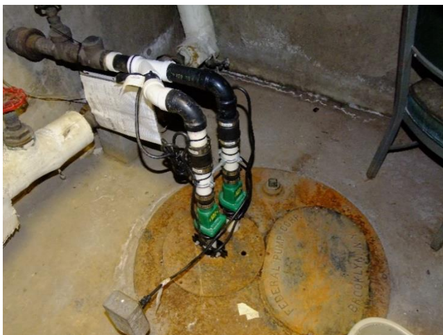
Figure 14: Sump Pump System
