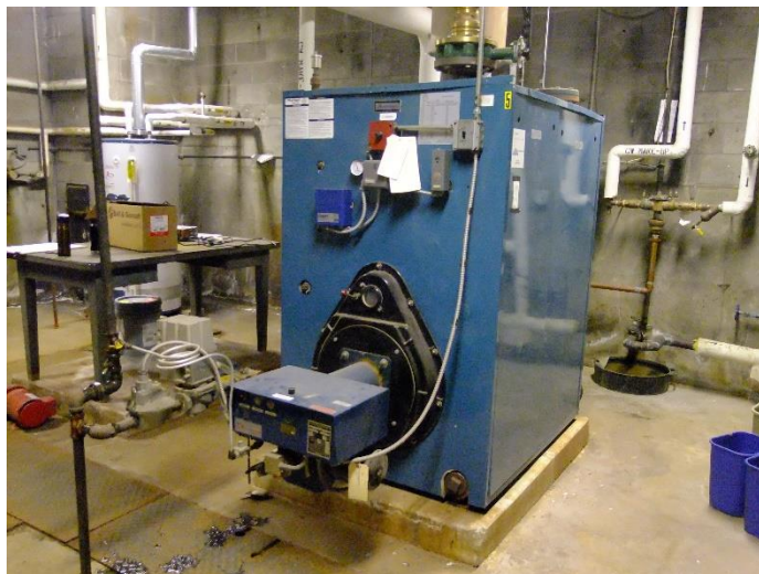
Figure 8: Central Gas-Fired Boiler Unit
