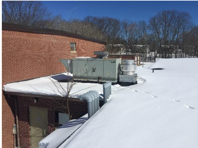
Figure 10: Rooftop Air Handler and Exhaust Fan (Typ.)
