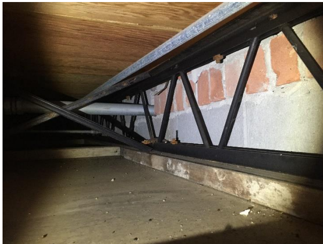
Figure 3: Open-Web Steel Truss System (Typ.)
