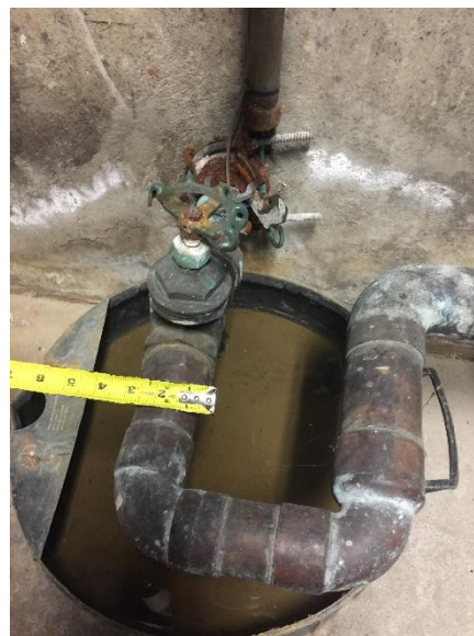
Figure 13: Main Water Service
