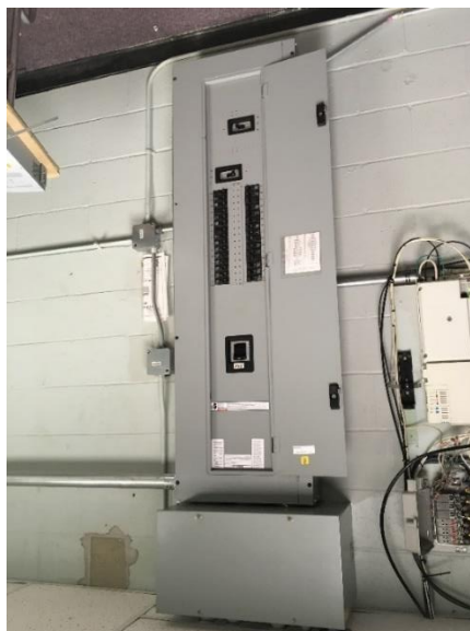
Figure 11: Main Circuit Panel
