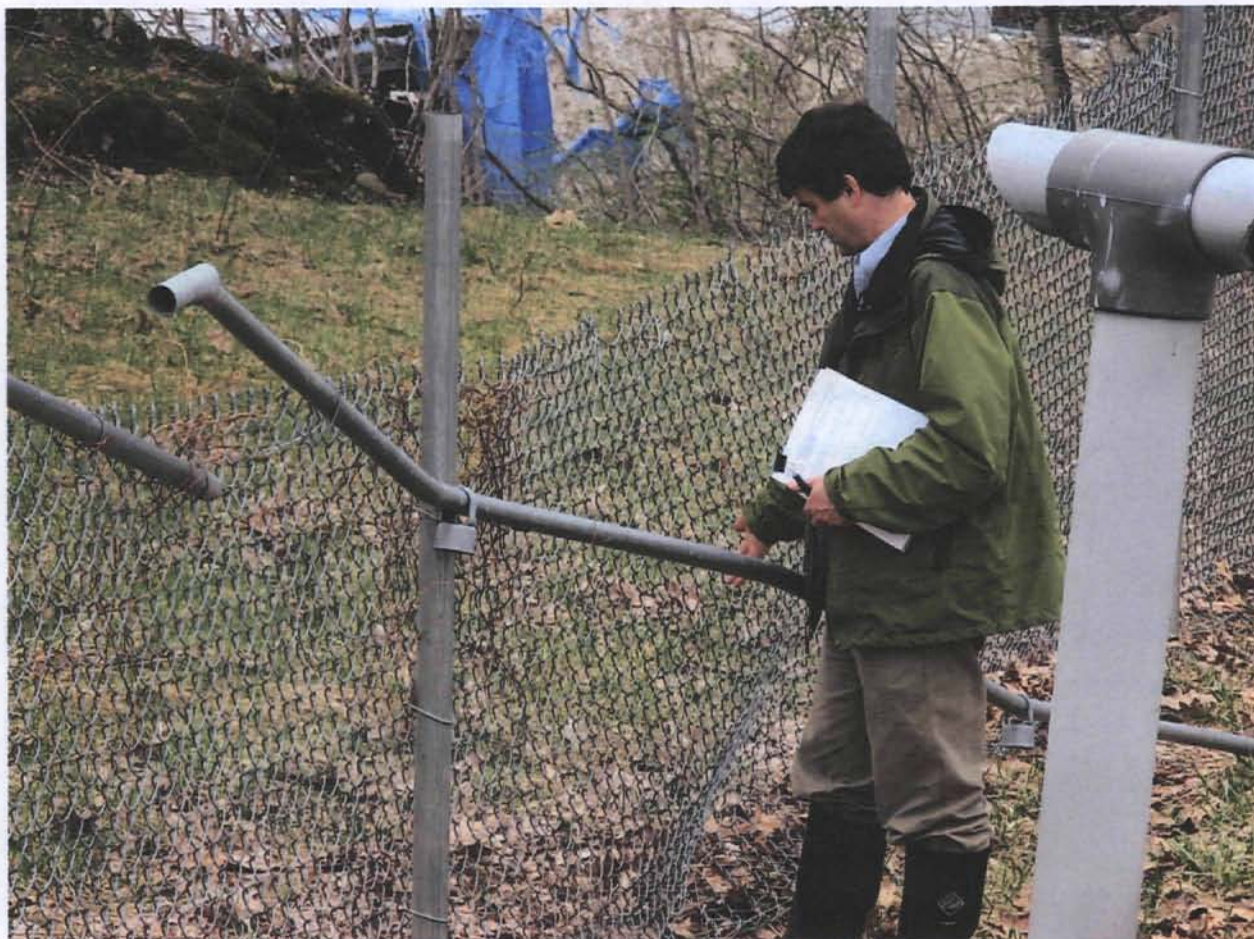
Figure 9. South-eastern section of fence showing snowstorm/ice damage
