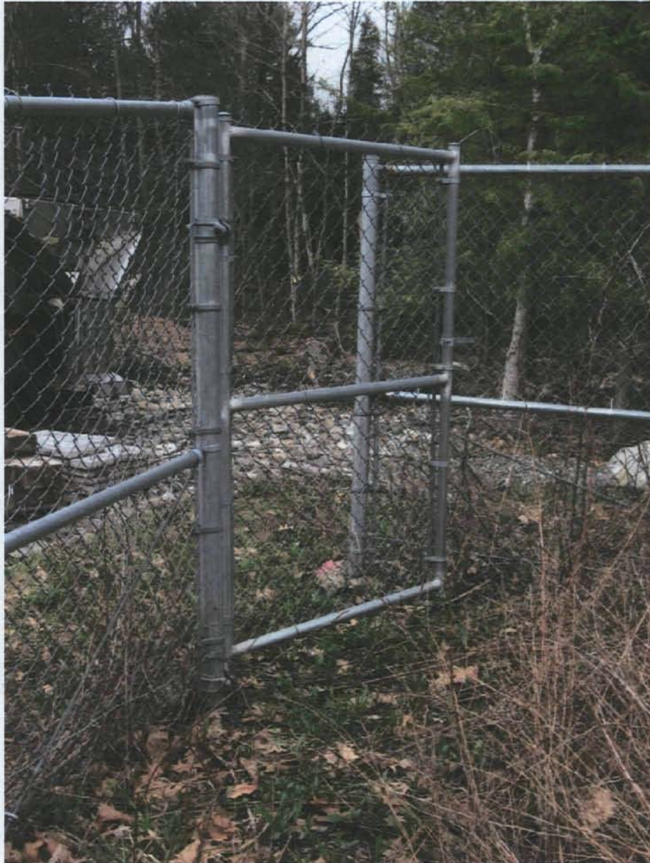
Figure 19. View of pedestrian gate at the southwestern corner of the fence unlocked, open and without a sign.
