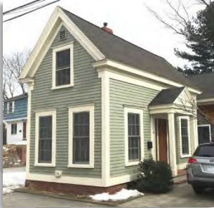
FHS/BAS/UBM Eaves can cut the bottom half of the window
