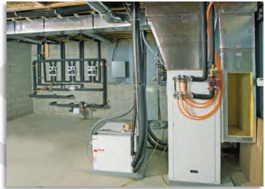
Geo-Thermal System in basement
