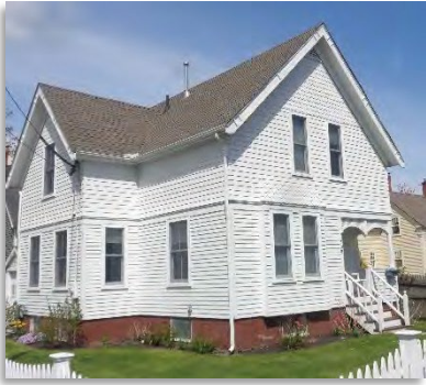
TQS/BAS/UBM Eaves fall at the middle of the window + turn in the roof.
