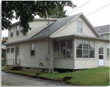
EAF/BAS/UBM Attic + dormer
