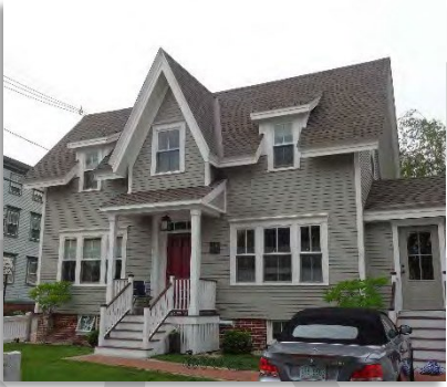
TQS/BAS/UBM Eaves cut through middle of window.
