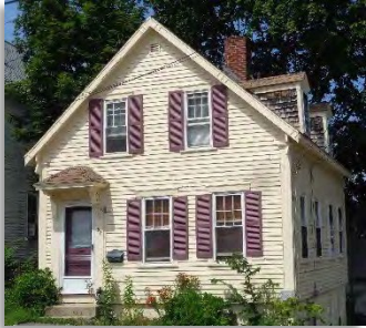
FHS/BAS/UBM Eaves at the bottom of window
