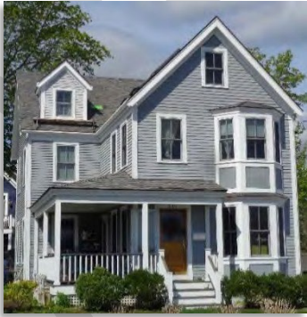
EAF/FUS/BAS/UBM Attic + turns in roof
