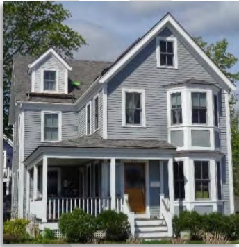
EAF/FUS/BAS/UBM Attic + turns in roof
