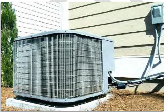
Heat pump (Mini-Split System)
