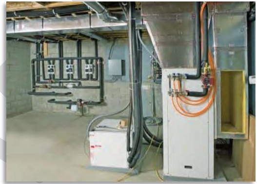
Geo-Thermal System in basement
