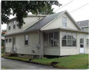
EAF/BAS/UBM Attic + dormer
