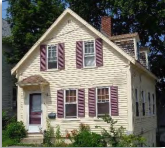
FHS/BAS/UBM Eaves at the bottom of window
