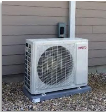
Heat pump (Mini-Split System)
