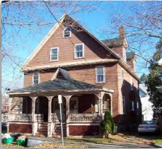
FAT/FHS/BAS/UBM Eaves at bottom of window, but another floor above.
