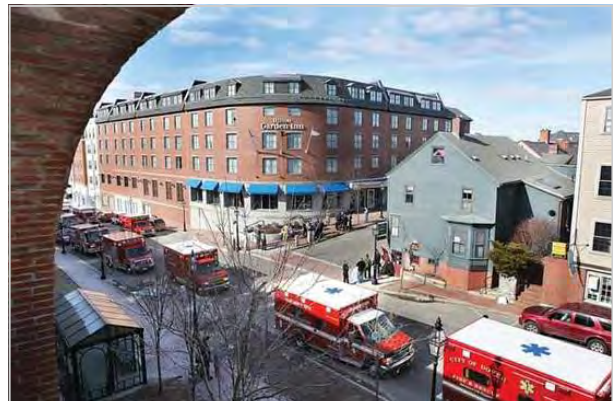
Mass casualty response to Feb. 15, 2010, carbon monoxide leak Photo courtesy of Seacoast Media Group
