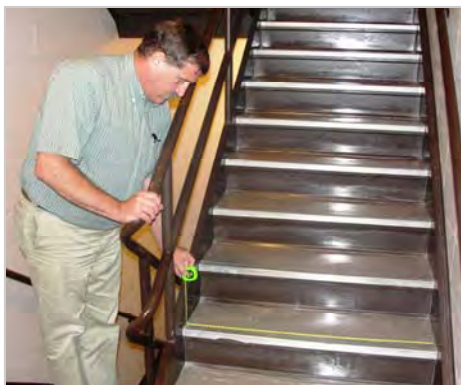
Assistant Building Inspector Roger Clum checks a staircase for code compliance
