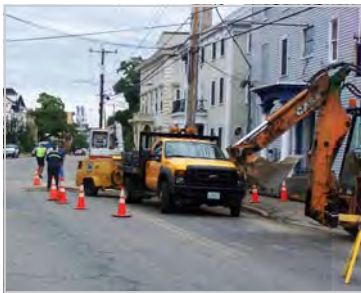
Islington Street roadwork
