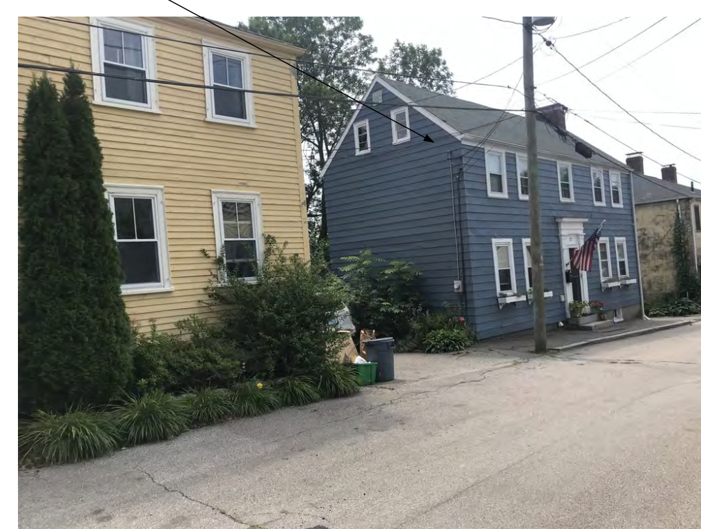
View looking S-W @ 52 Prospect Street
