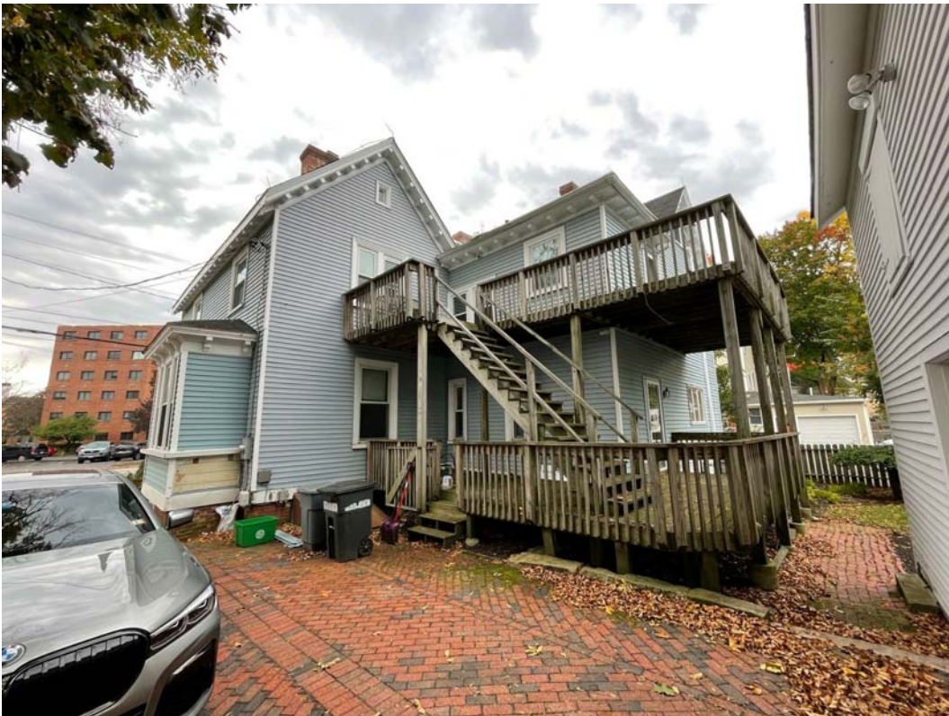
IMAGE OF RIGHT SIDE AND REAR ELEVATION
