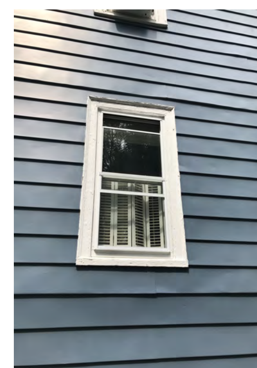
Existing Casing @ Rear Elevation
