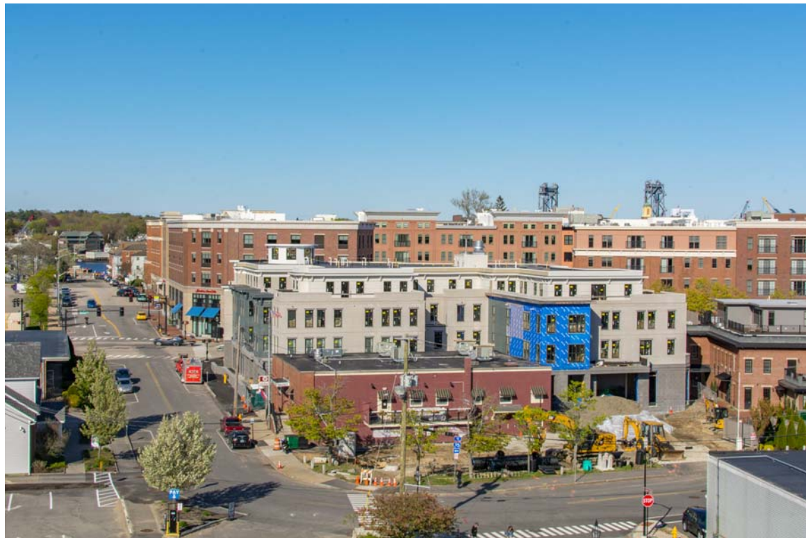
EXISTING PICTURE FROM FOUNDRY GARAGE ROOF
