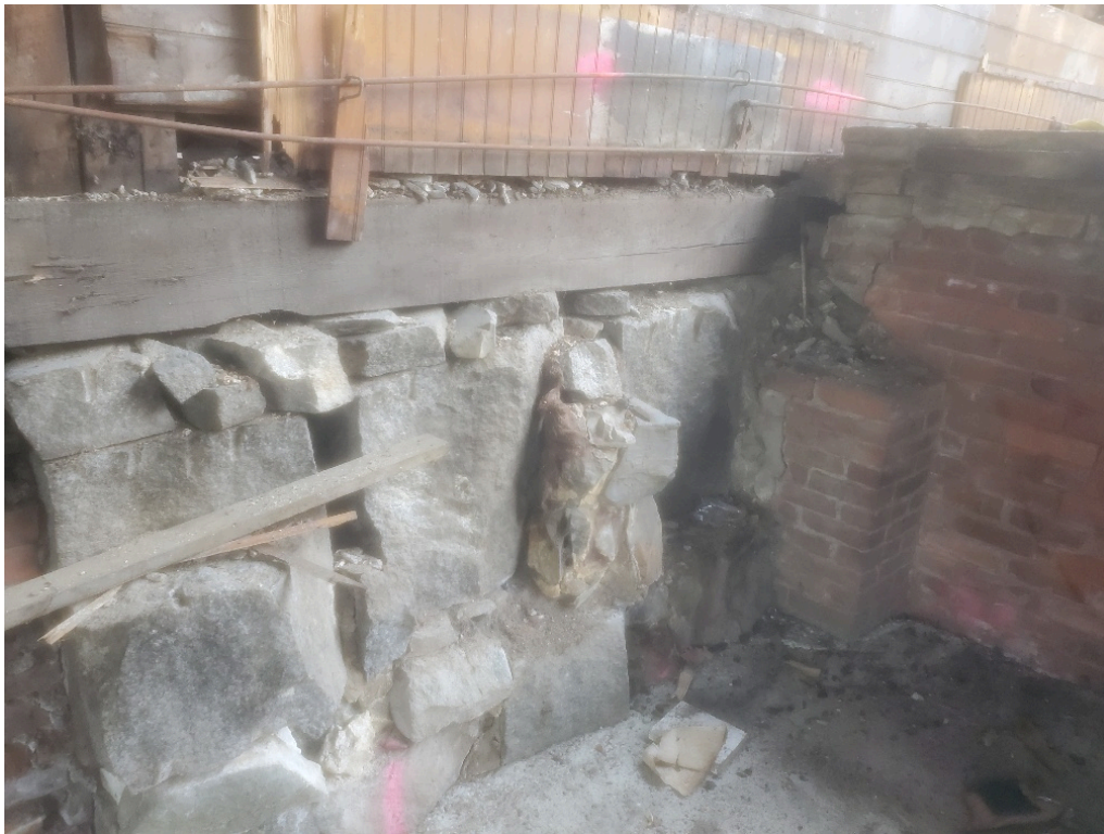
202 COURT STREET – EXISTING ROCK-RUBBLE FOUNDATION
