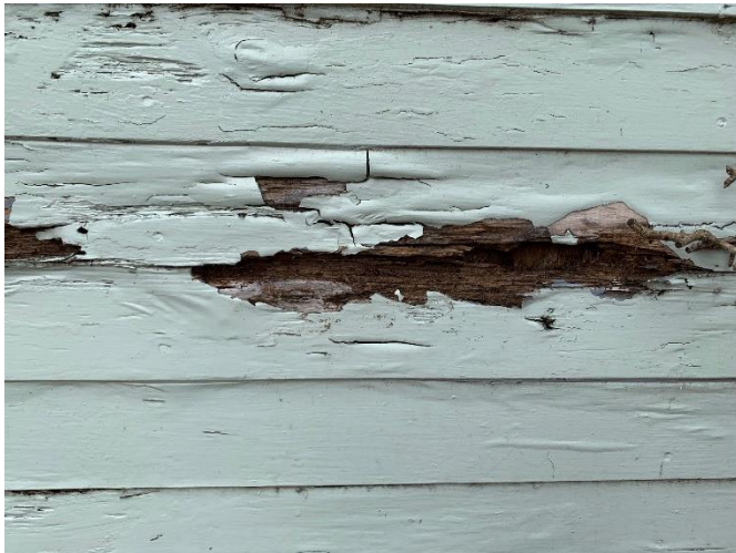
Extensive rot in rear siding penetrating into shed foundation
