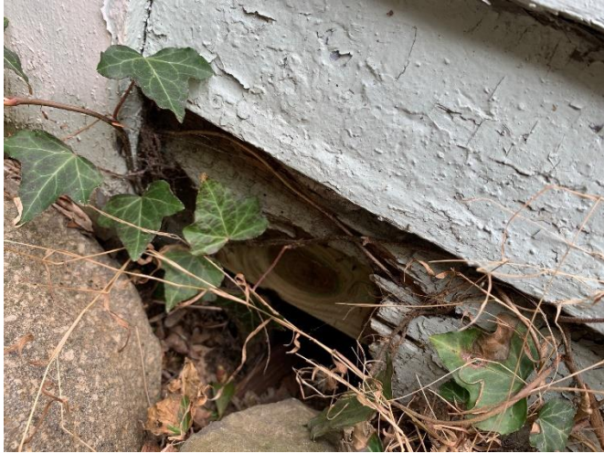
Rot in base of corner post through to subfloor with no remaining exterior support for post
