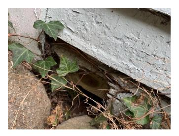
Rot in base of corner post through to subfloor with no remaining exterior support for post
