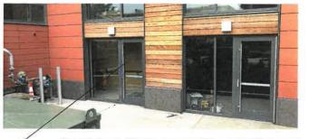
C. Door relocated from left to right side of storefront bay. Exit corridor ramps up from the garage level and the door had to flip to accommodate the ramp.
