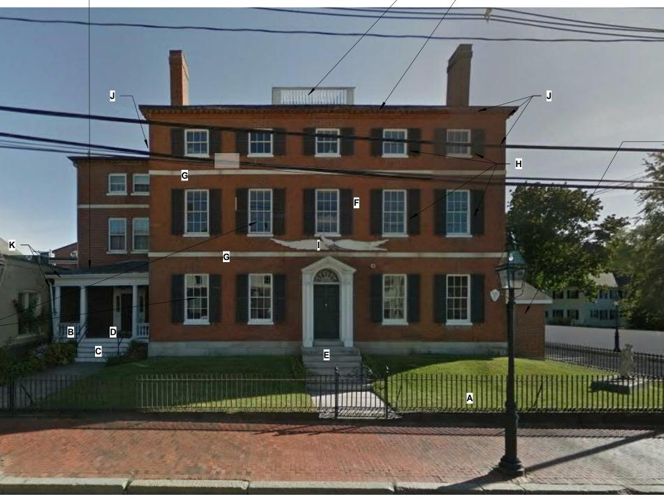
ONE STORY BUILDING ADDITION TO BE DEMOLISHED. EXTERIOR **BRICK OF MAIN BUILDING** TO BE REPAIRED AND **REPOINTED AS** REQUIRED.
