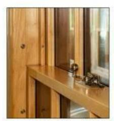
The checkrail detail above highlights the concealed spiral balances of this unit which allows only the beauty of wood to be seen.
