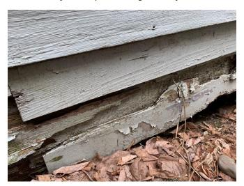
Collapse of subfloor visible from exterior rear of shed
