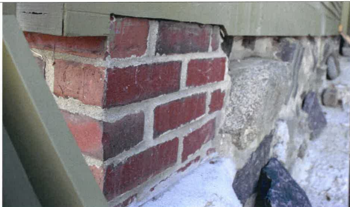
INSERT # 12. Front right (northwest) corner top of the foundation along the right (West) side of house, showing the brick foundation replacement was only done at the front
