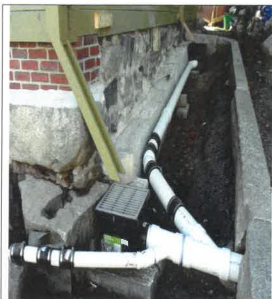
INSERT # 2 Completed roof rainwater drainage system at right/West side of house
