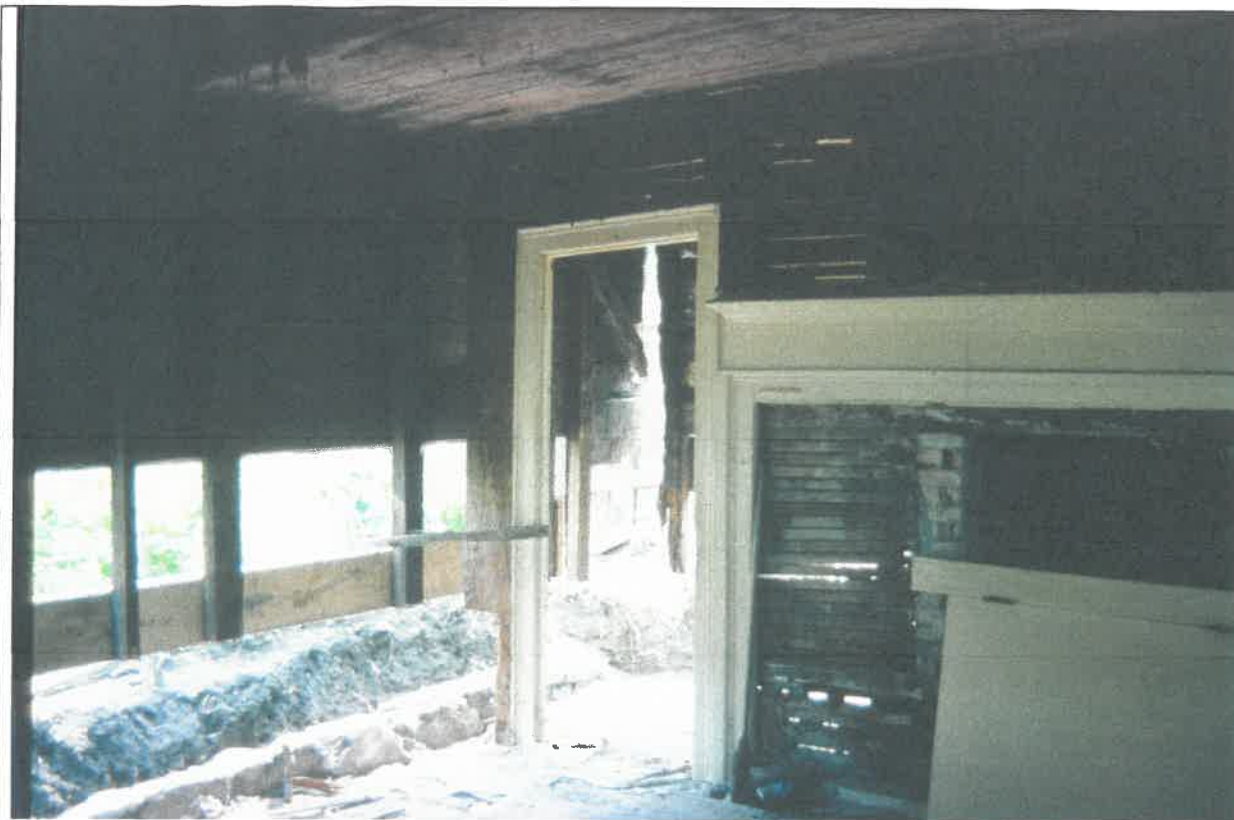
40 Howard St. 1985, during renovations. Interior, first floor photo, showing left side (East) at rear (South) of house – revealing top of foundation below grade.
