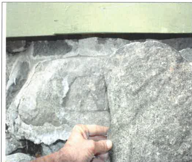
INSERT #30 Ledge sample held next to existing foundation to show similar character
