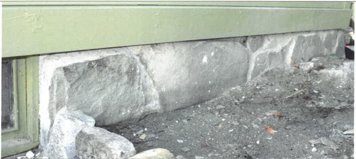
INSERT #43 Existing stone veneer over concrete foundation added in 1980s. Right side (West ) at rear of house. The 2-inch veneer is comprised of ledge and flagstone in this section
