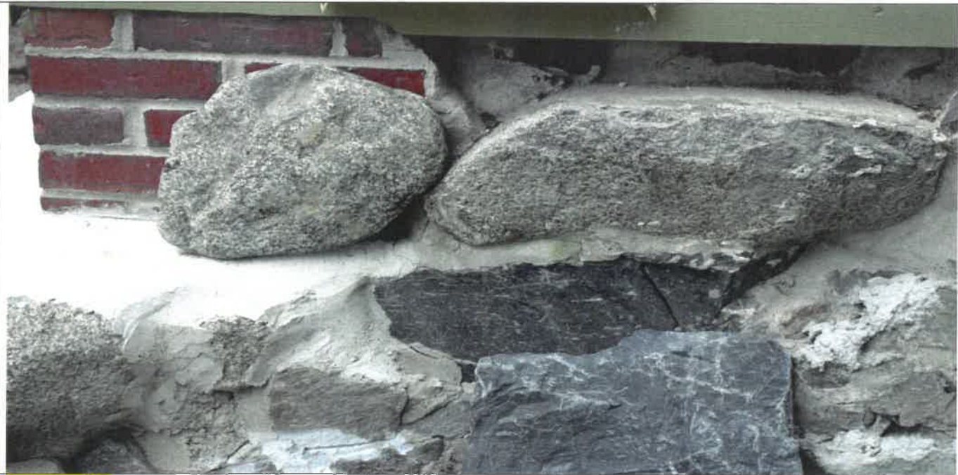
INSERT #37 Matching granite sample (above left) and bluestone sample (below center), dry-laid
