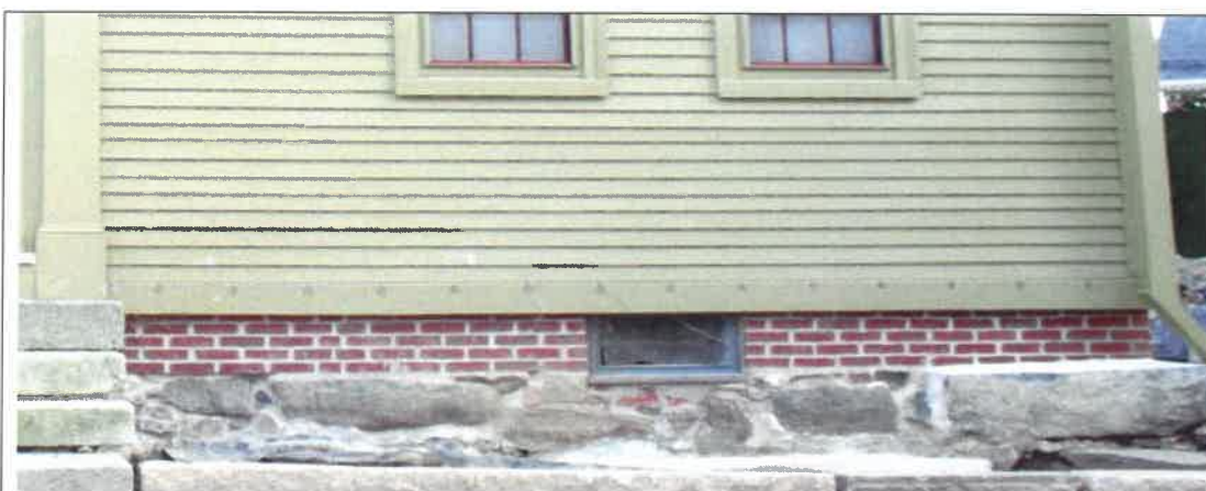
INSERT # 10. Close up of foundation exposed after drainage system installation
