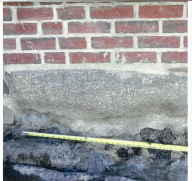
INSERT #20 original 30 inch granite stone in front (North) foundation
