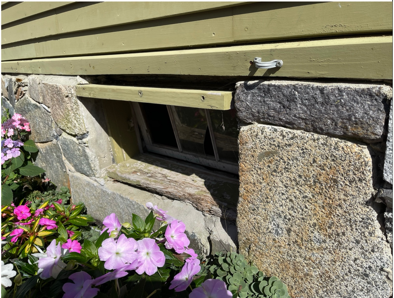
Exhibit-4 current stone veneer foundation and basement window (with ill-fitting water table trim board, addressed below)
