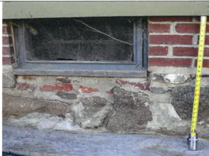
INSERT #26 The average height of the above-grade foundation is 22-27 inches
