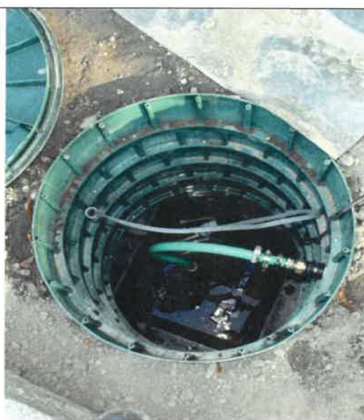
INSERT # 3 5-foot deep catch basin for French drain-type system under future garden
