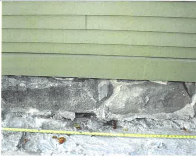
INSERT #22 Large original granite and ledge stones in right side (West) foundation
