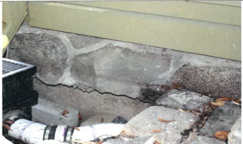
INSERT #42 Existing stone veneer at rear corner (Southwest), with 2-inch granite, and flagstone over concrete foundation
