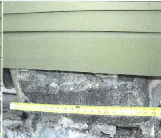
INSERT #23 original 20 inch granite stone in right side (West) foundation
