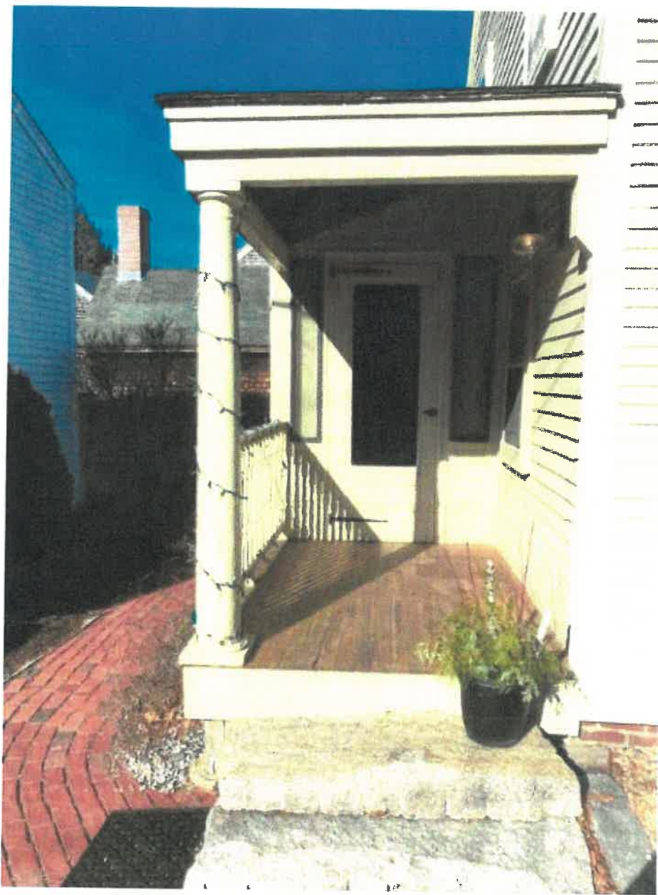
Existing Porch Entrance with 30" Door South entrance
