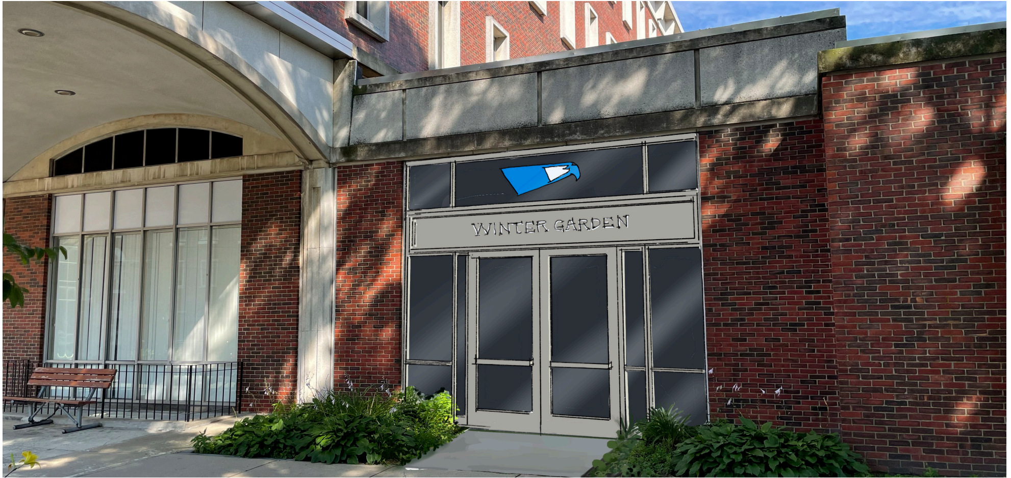
Winter Garden entrance view from Daniel Street
