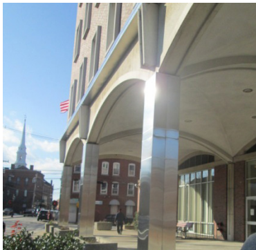
Stainless Steel-Clad Columns on Daniel Street.
