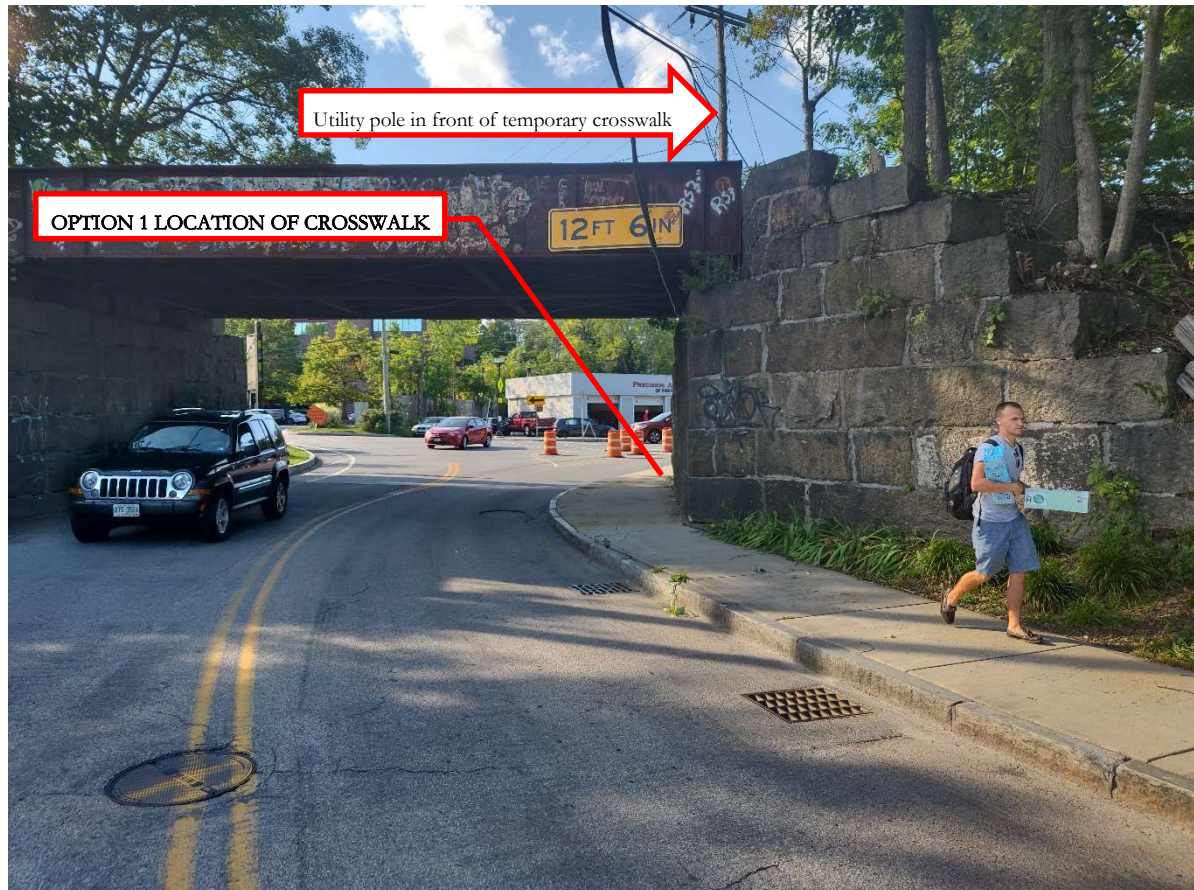
Photo 2: Looking north under the Railroad overpass along Bartlett Street toward the intersection for the 90-ft stopping sight distance point
