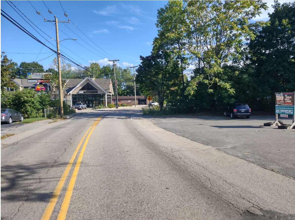
Photo 3: Looking south along Bartlett Street toward the Option 2 cross walk location from the 148-ft sight distance location. As can be seen the trees would need to be limbed up
