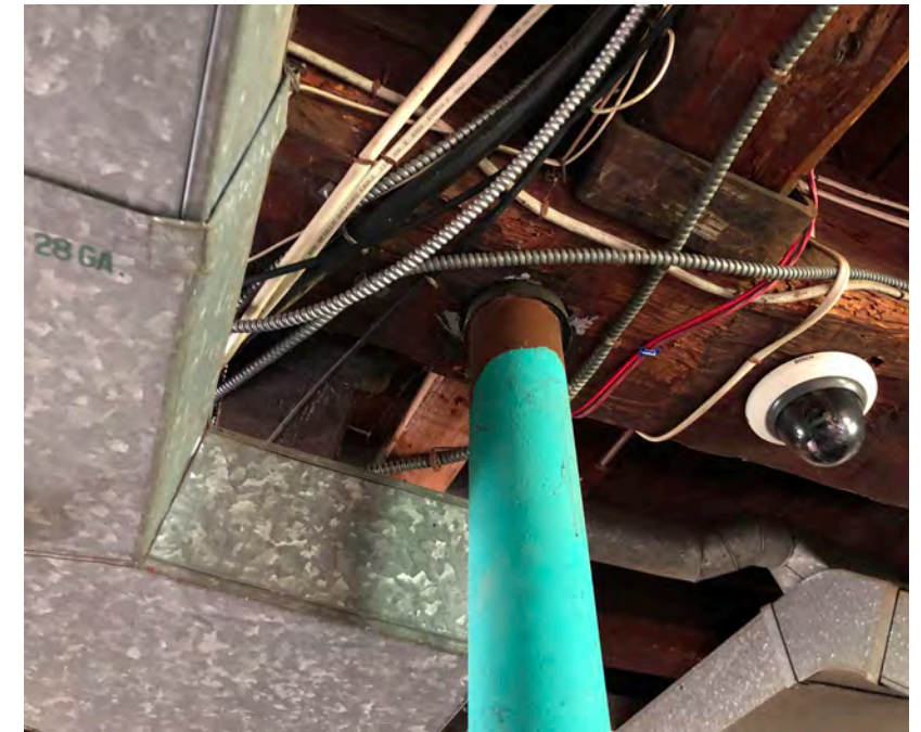
Shaw 1st Floor - Steel Support Post
