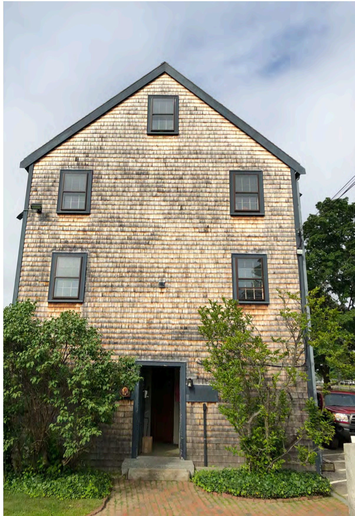
West Elevation - Entrance to building
