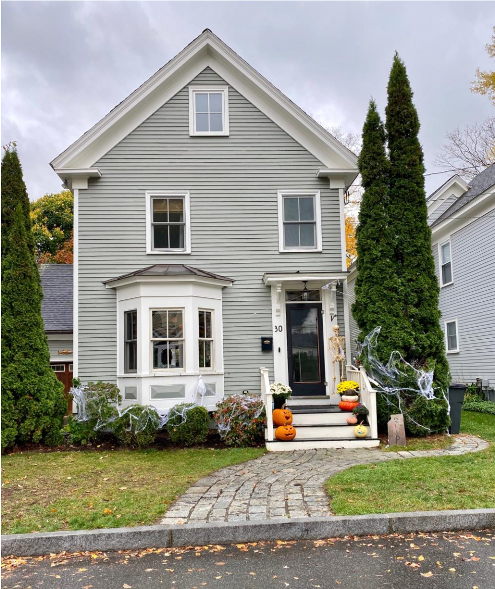
30 Spring Street - Exterior Photos.
