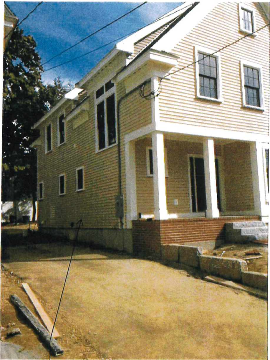
Northerly Side of House
