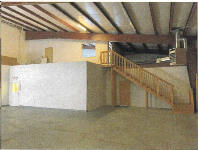
View to 2 nd Floor
