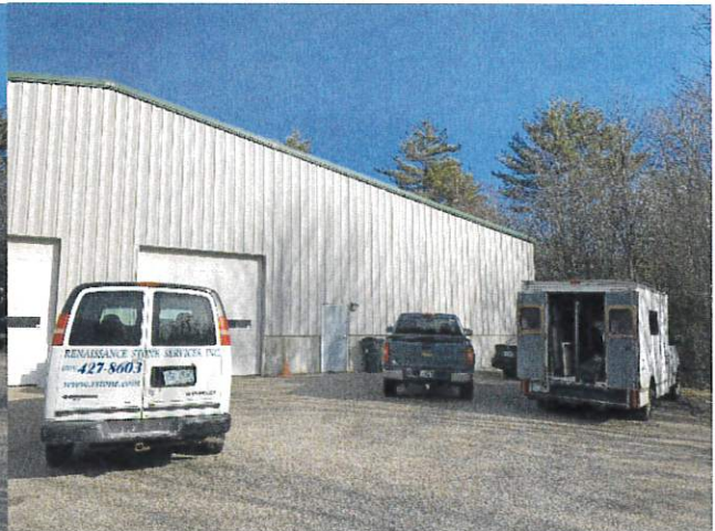
Rear View of 6A Parking Area
