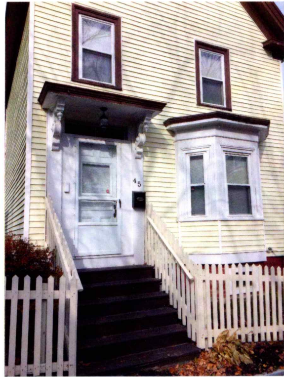
VEWS OF EXIST FRONT STEPS
