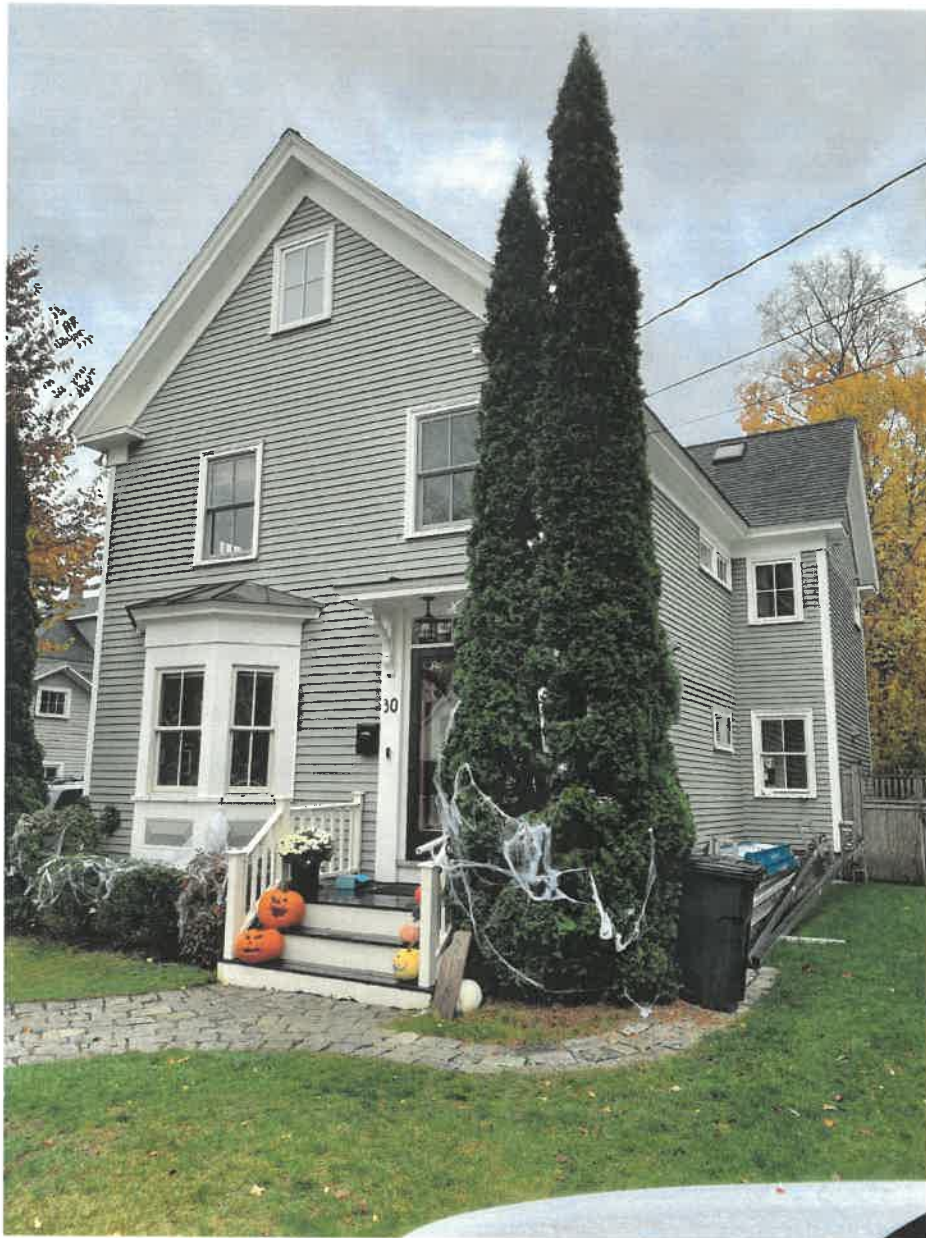
The right side of the porch would end just past the existing arborvitae, and would not exceed the width of the back half of the house.
