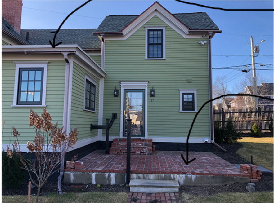
VIEW FROM DRIVEWAY
