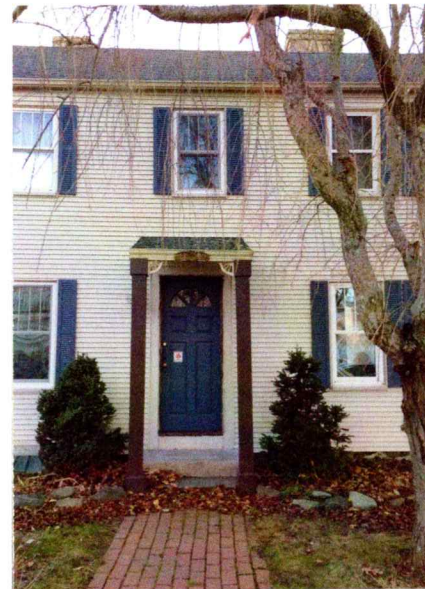
EXIST FRONT DOOR
