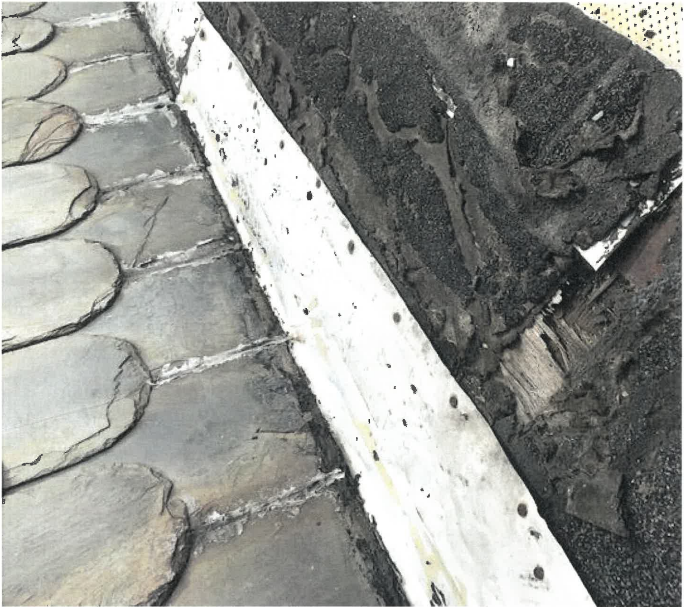
Images of appearance of rubber membrane roof:
