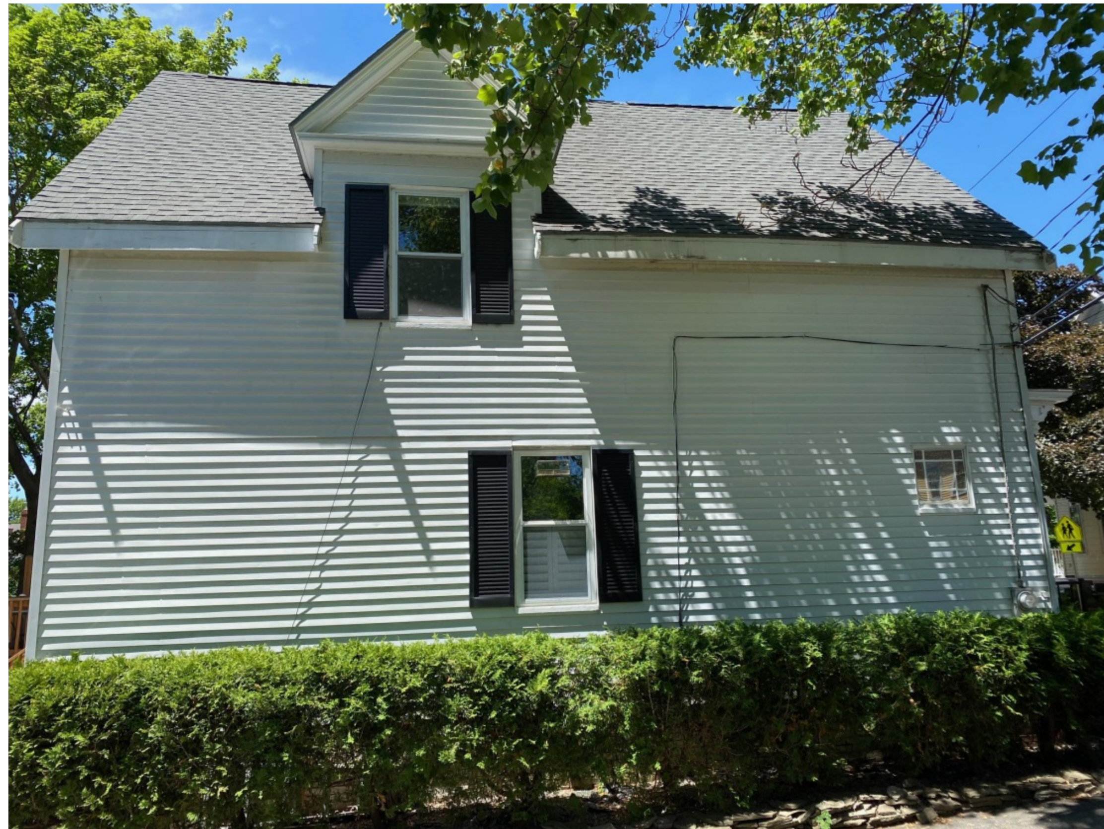
LEFT ELEVATION PHOTO | SIDEVIEW
