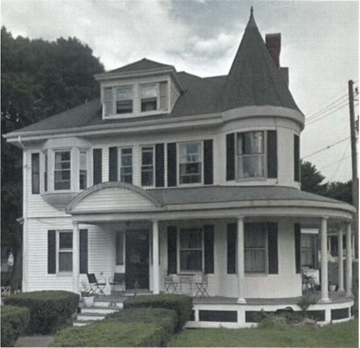
169 Lafayette Road, Portsmouth, New Hampshire Porch Roof BEFORE renovation
