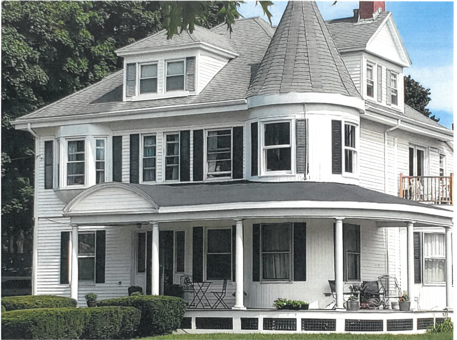
169 Lafayette Road, Portsmouth, New Hampshire Porch Roof AFTER renovation
