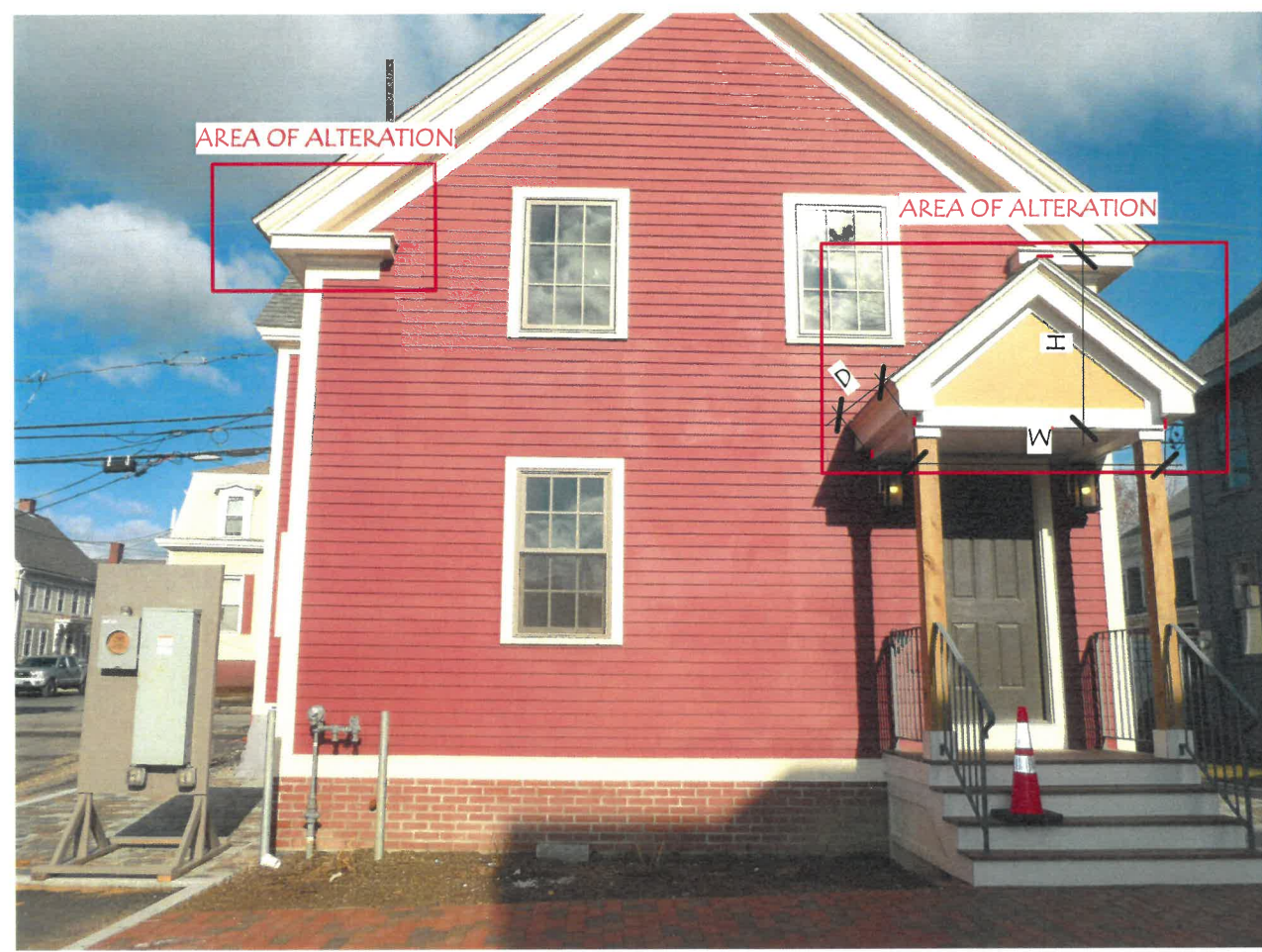
412 SOUTH ELEVATION- AS BUILT
