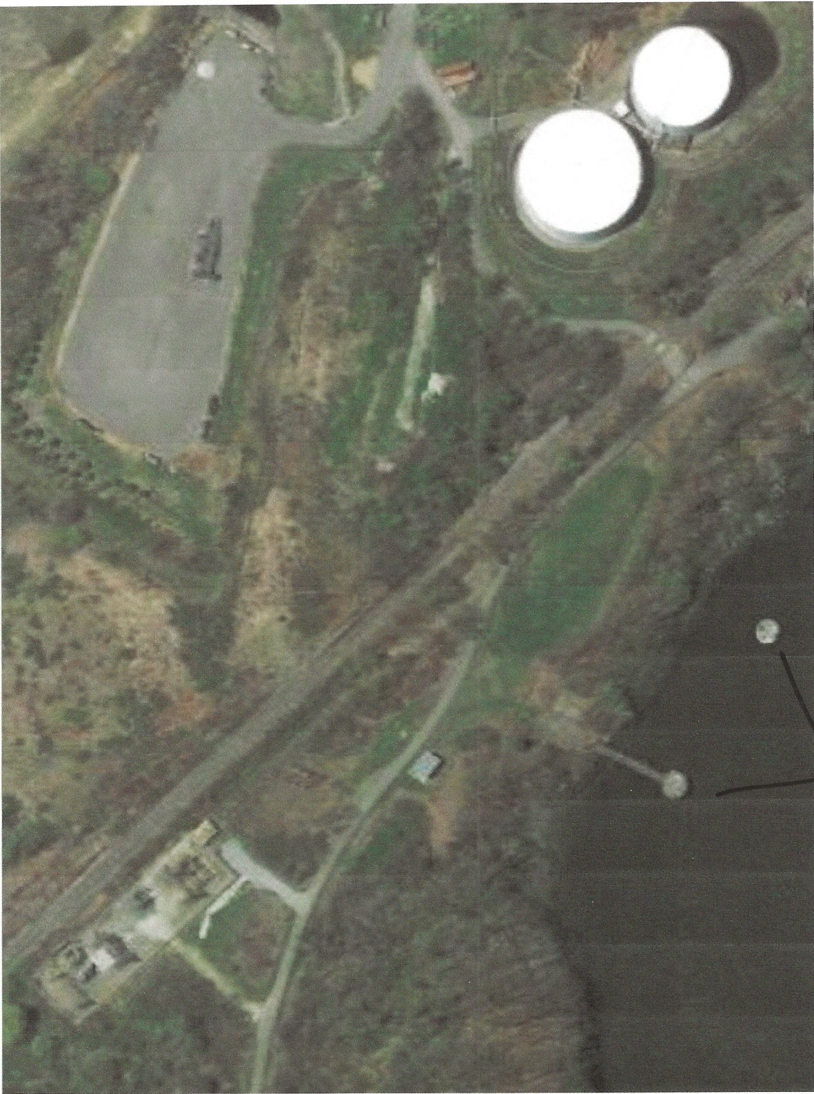
Jacobs Wharf and Mooring
