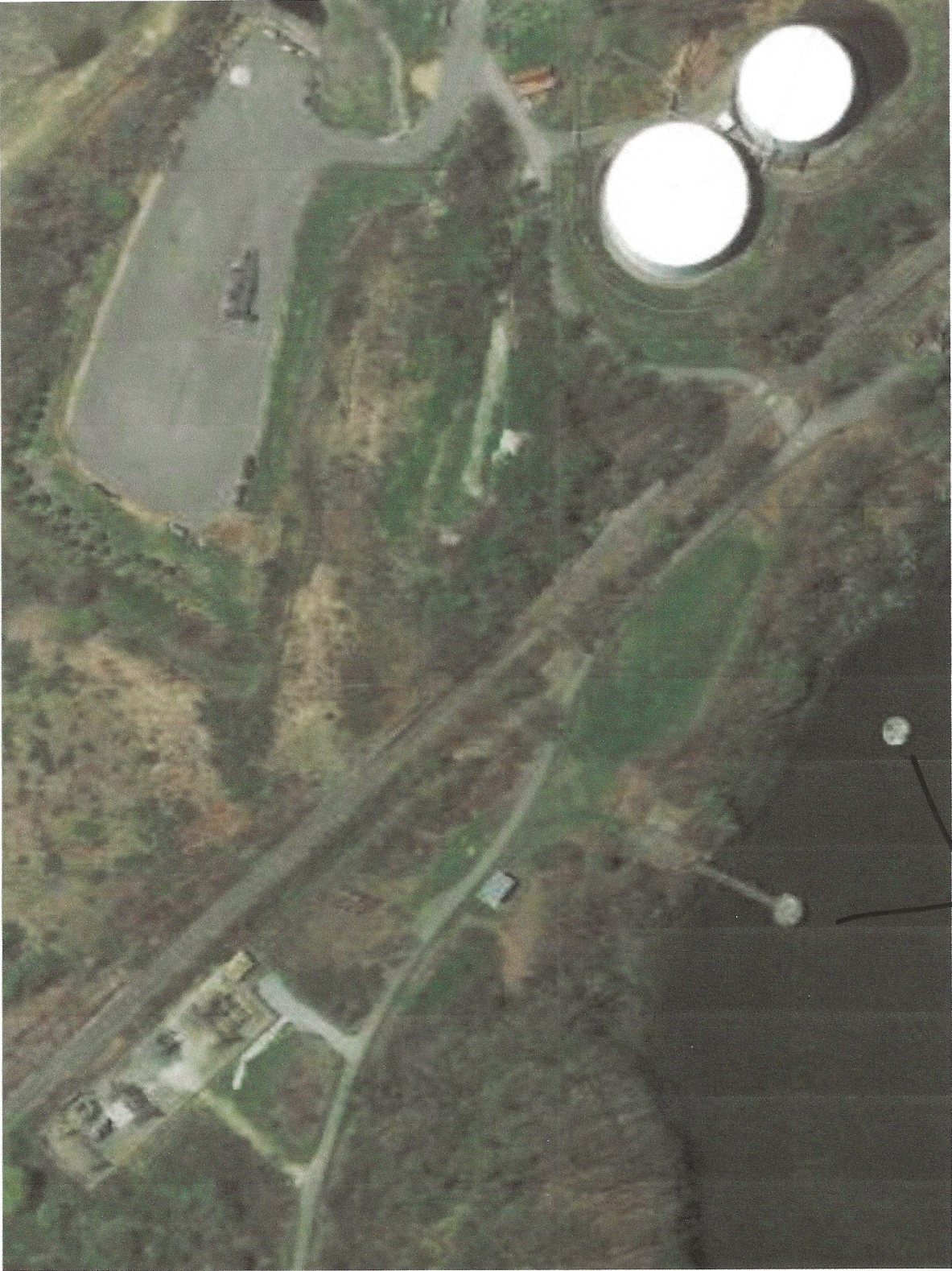
Jacobs Wharf and Mooring
