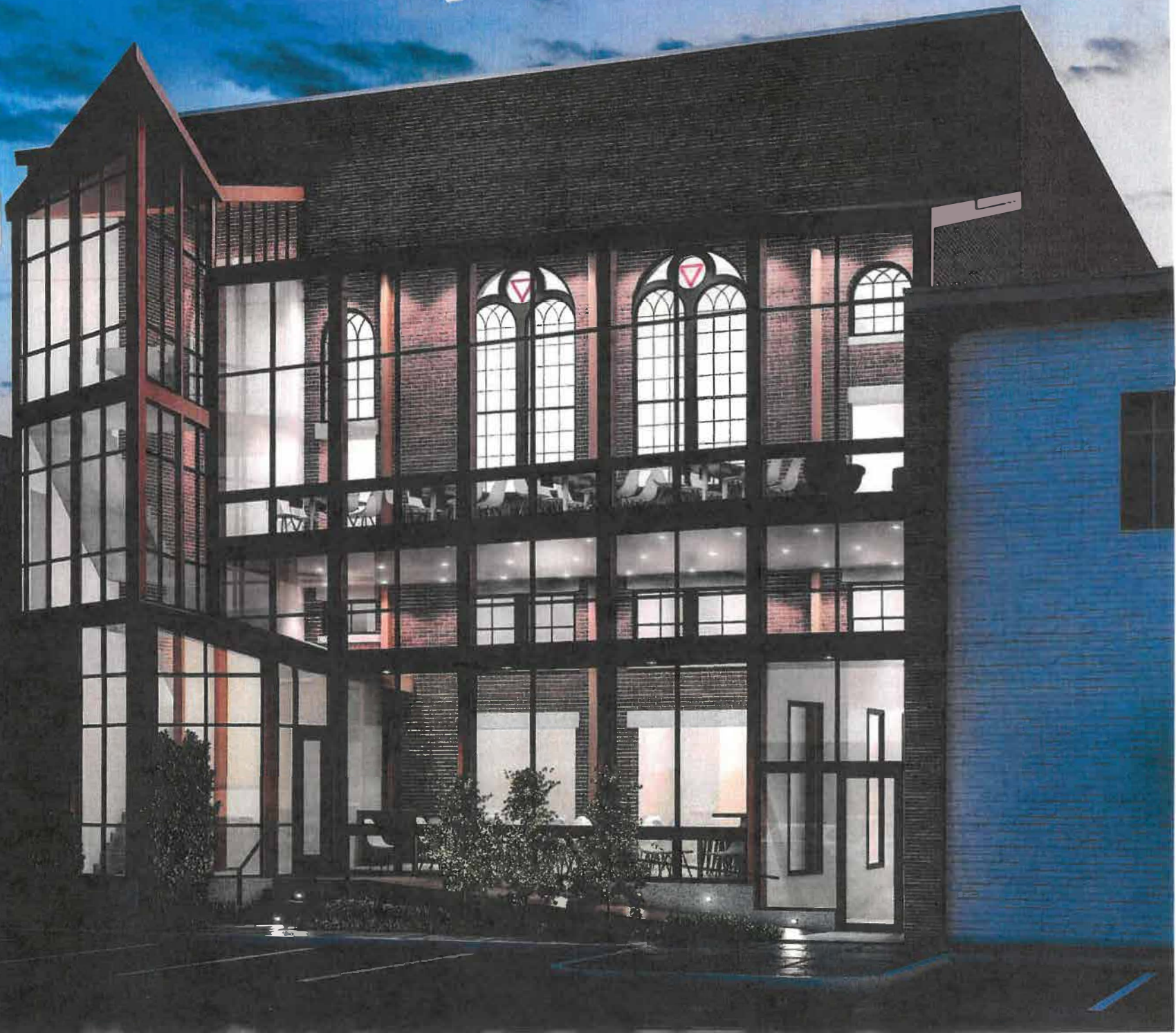
135 Congress Street Rear After Renovations
