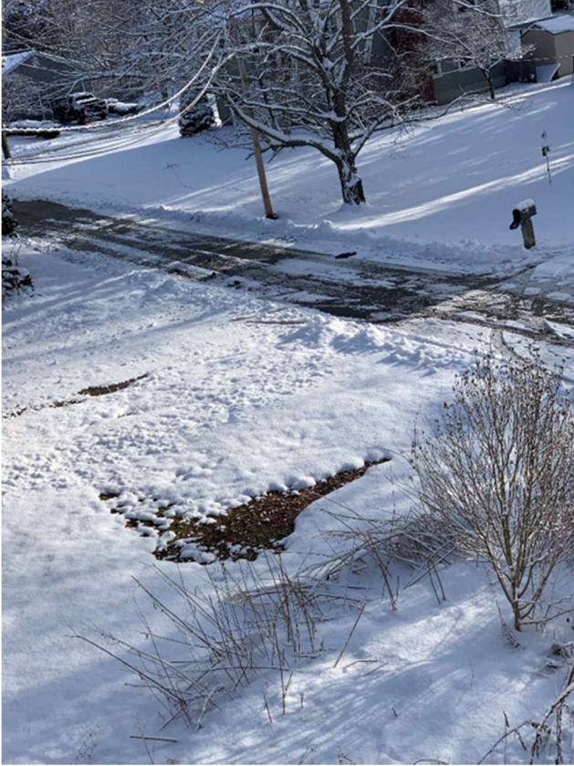
December 18, 2019 – visible water after snow between house and garage (66 Benson St)
