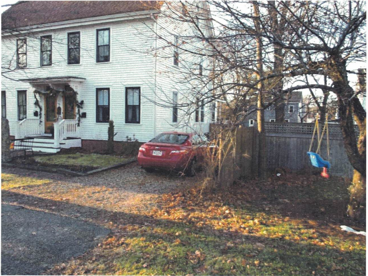
Right Front of Lot 23 (House Lot) from Thornton Street
