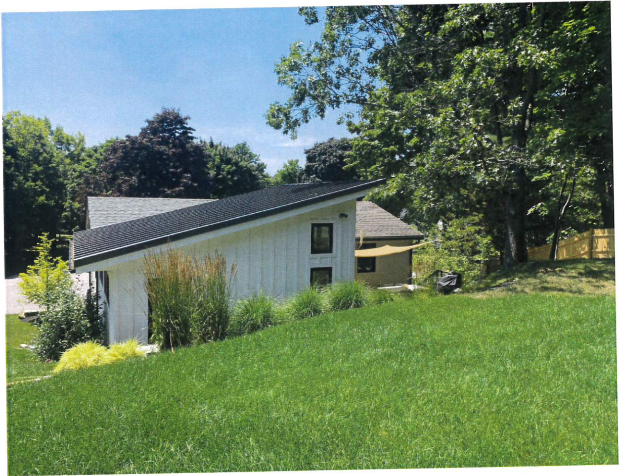
Rear-Left Elevation Picture
