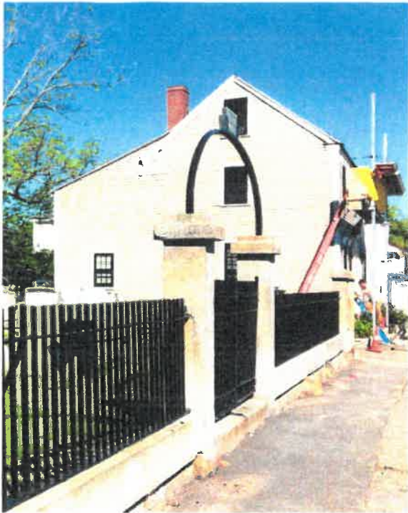
Existing Rear Shed Roof
