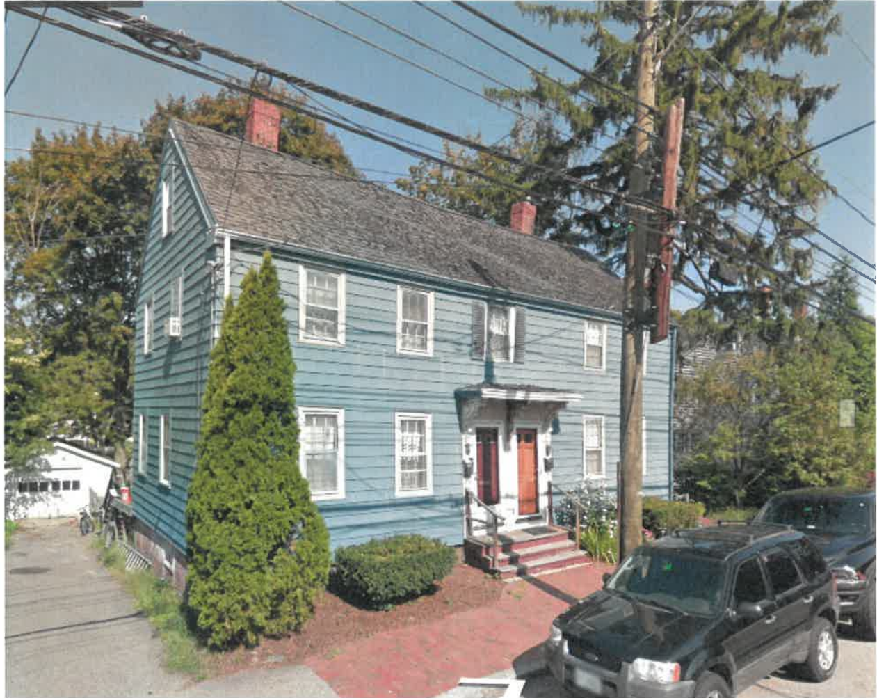
Existing Steps – 442 Middle Street
